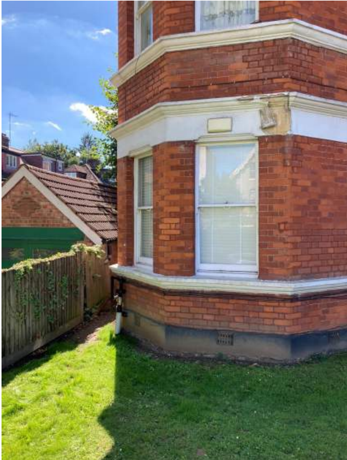
Figure 6 Installed pipework to the north elevation.
