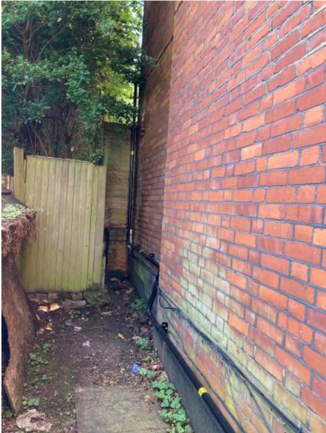
Figure 1 Installed pipework to the east elevation.
