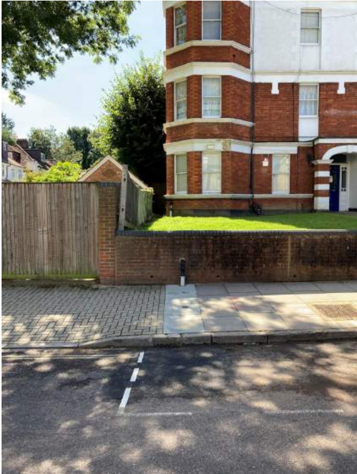
Figure 5 Installed pipework to the north elevation.
