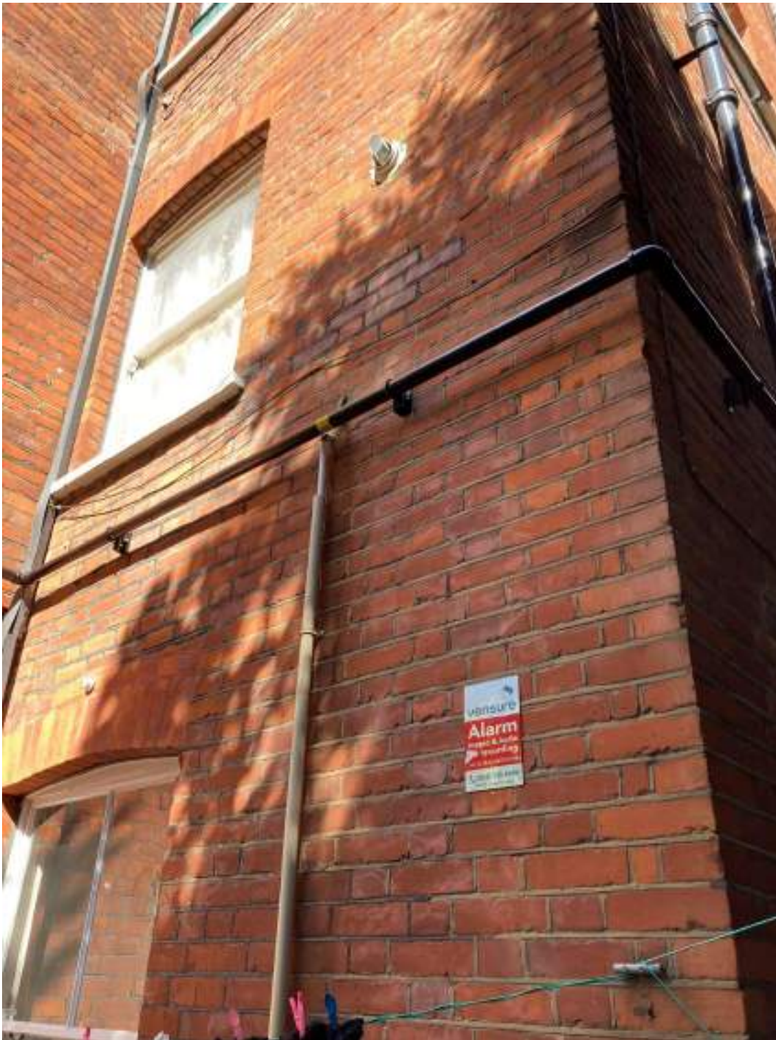
Figure 4 Installed pipework to the south elevation 2.
