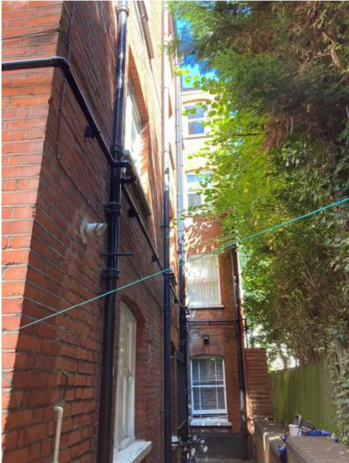
Figure 2 Installed pipework to the east elevation.
