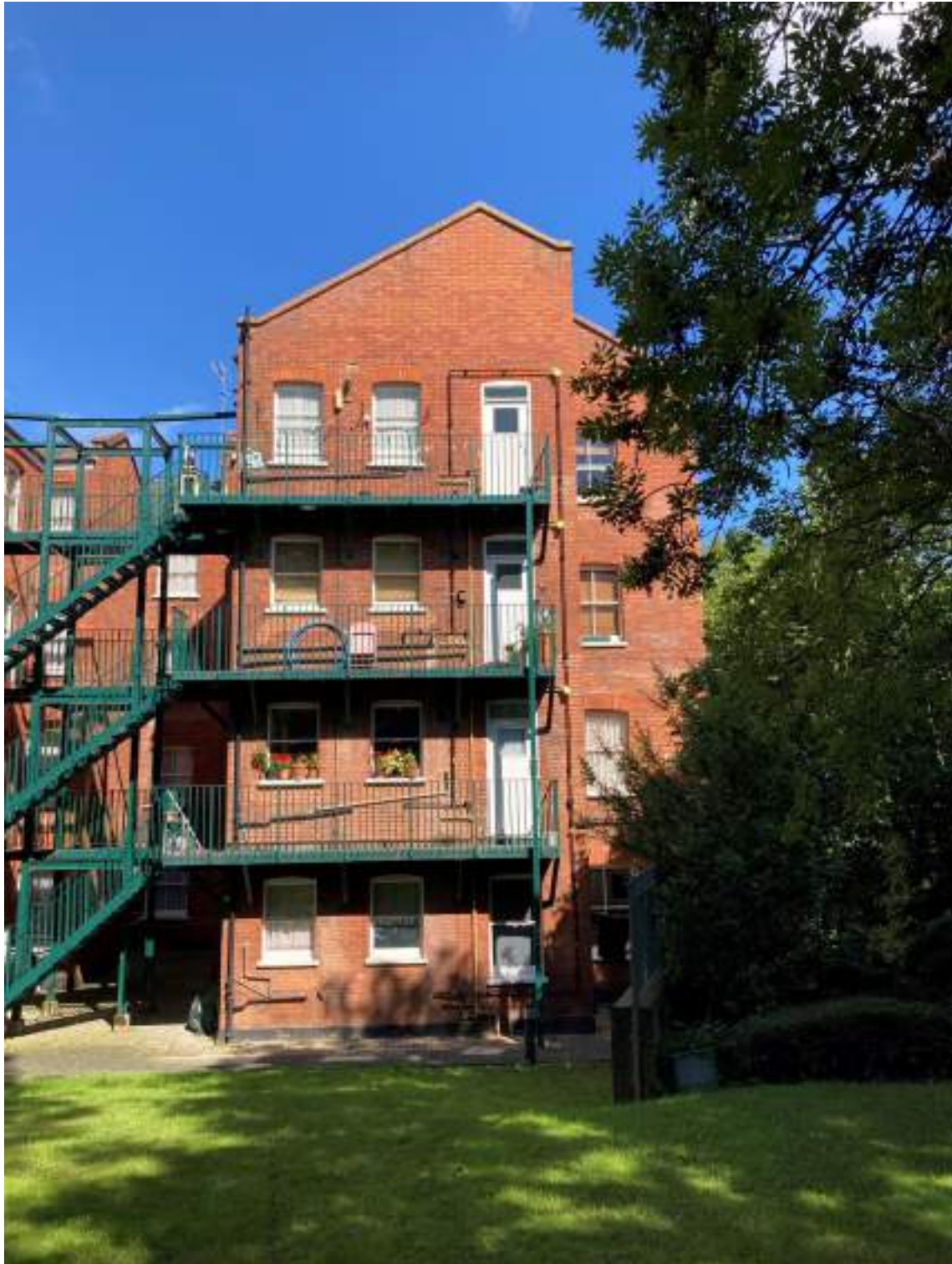
Figure 3 Installed pipework to the south elevation 1.
