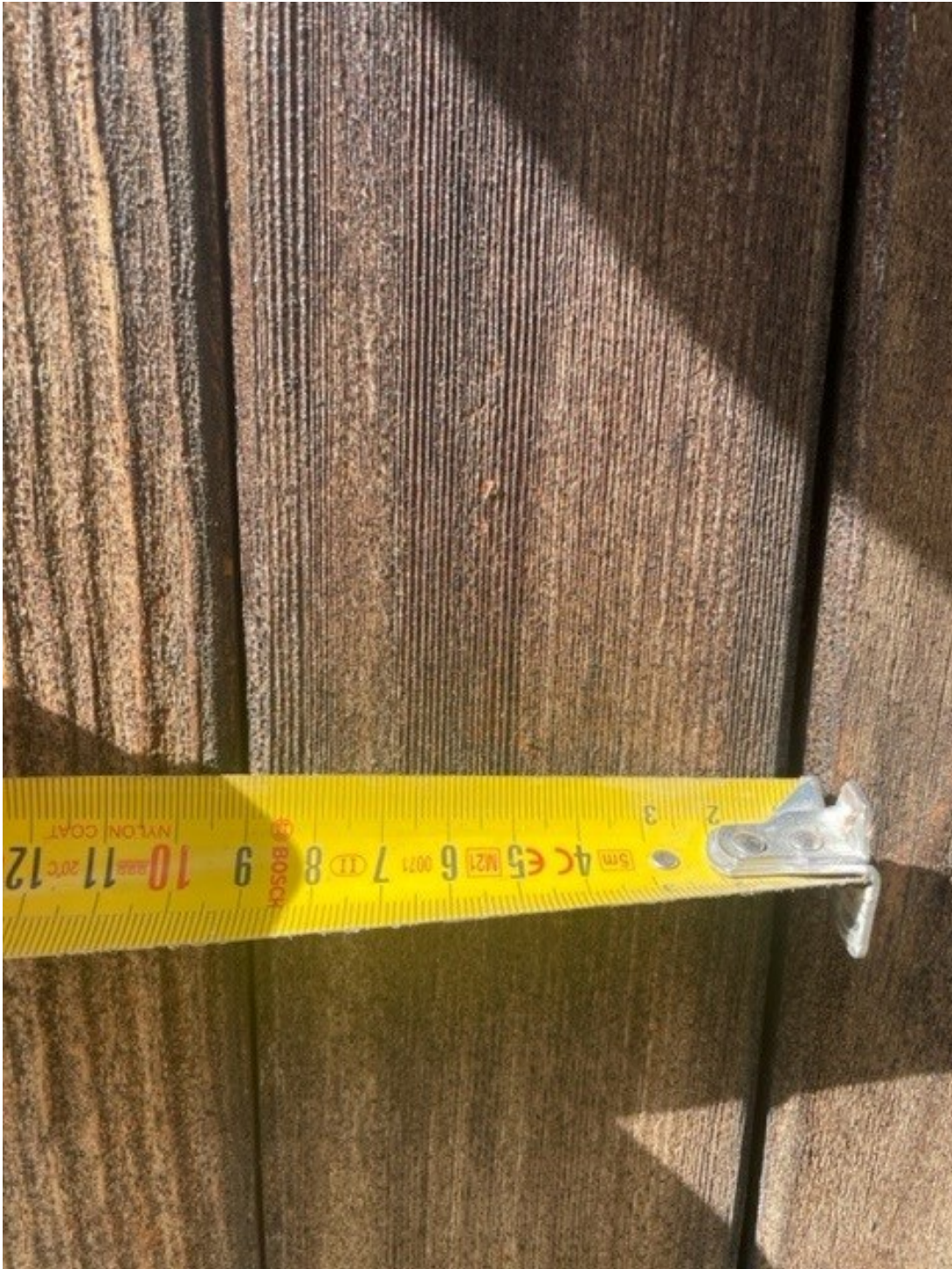
(b) close-up up view of existing cladding board with tape measure for scale.
