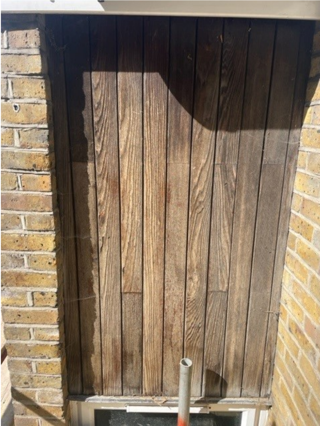
(a) full panel view of existing cladding.
