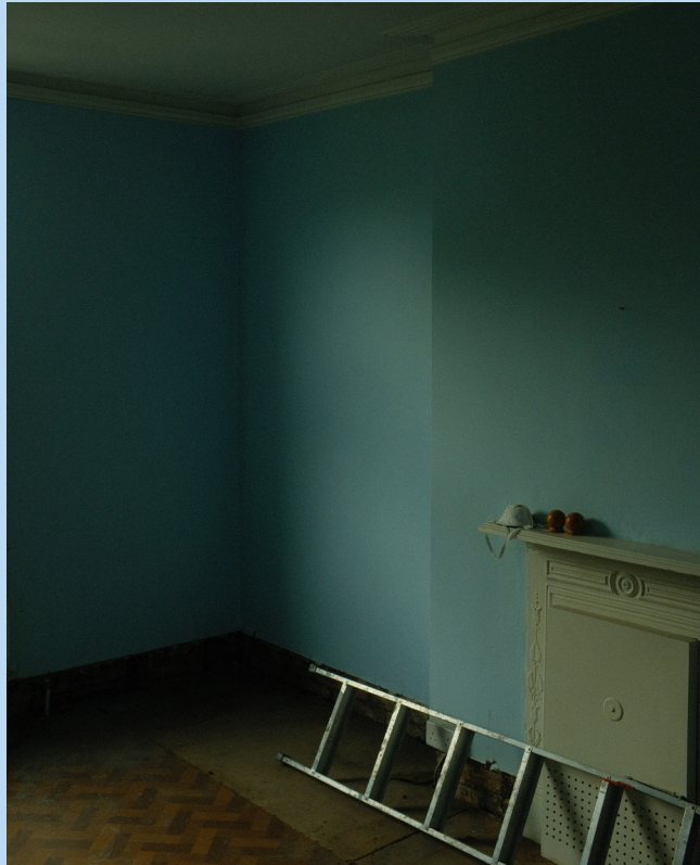
11 Lynmouth Rd - Chimney Breast Retained Internally.
