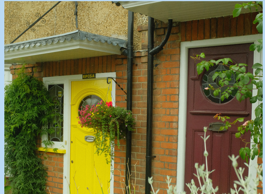
Lynmouth Rd - Entrance doors on building edge.
