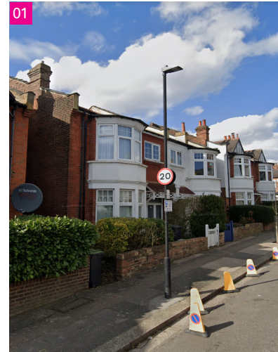
11 Lynmouth Road North Approach
