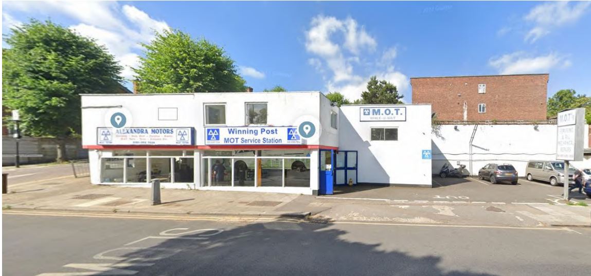
Photograph 2: Garage building externally
