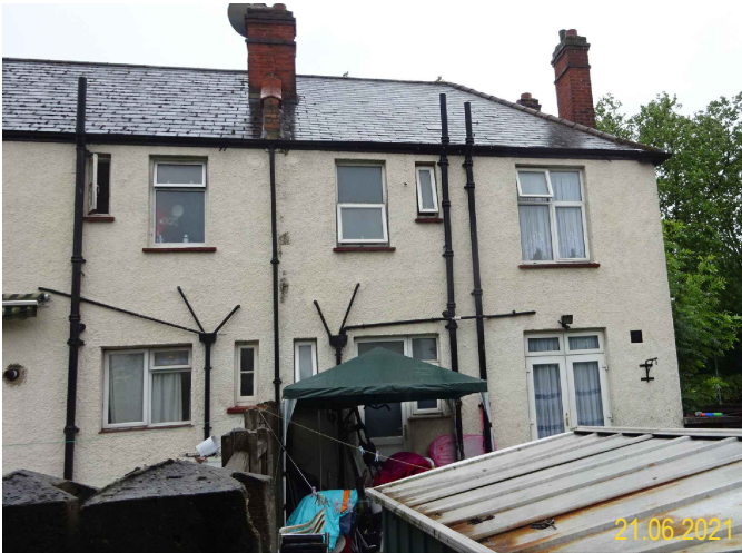
4.3 - View of the neighboring property at No.106 Downhills Park Road
