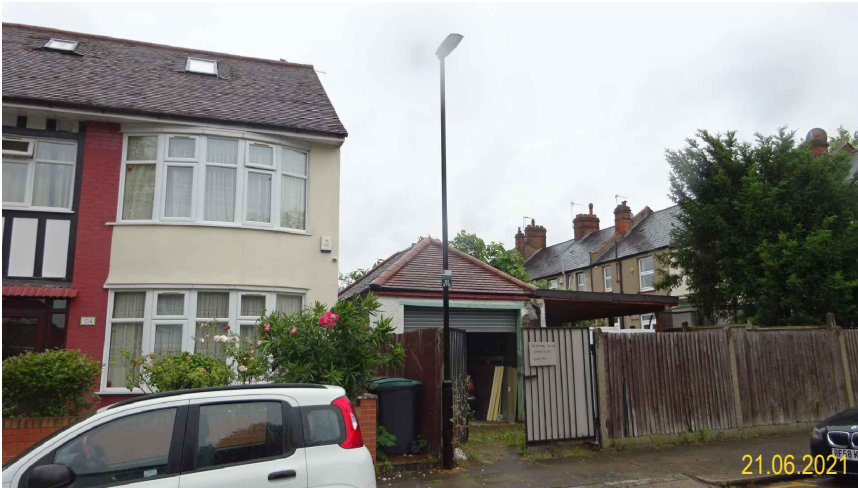
4.1 - View of the existing garage from Higham Road
