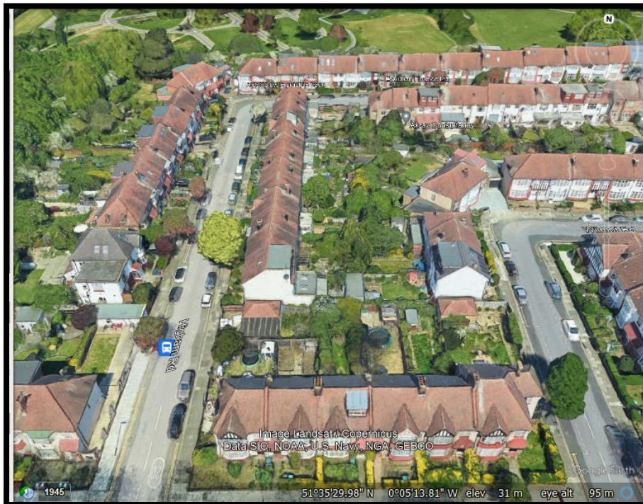
Figure 1 Aerial Photograph of Locality
