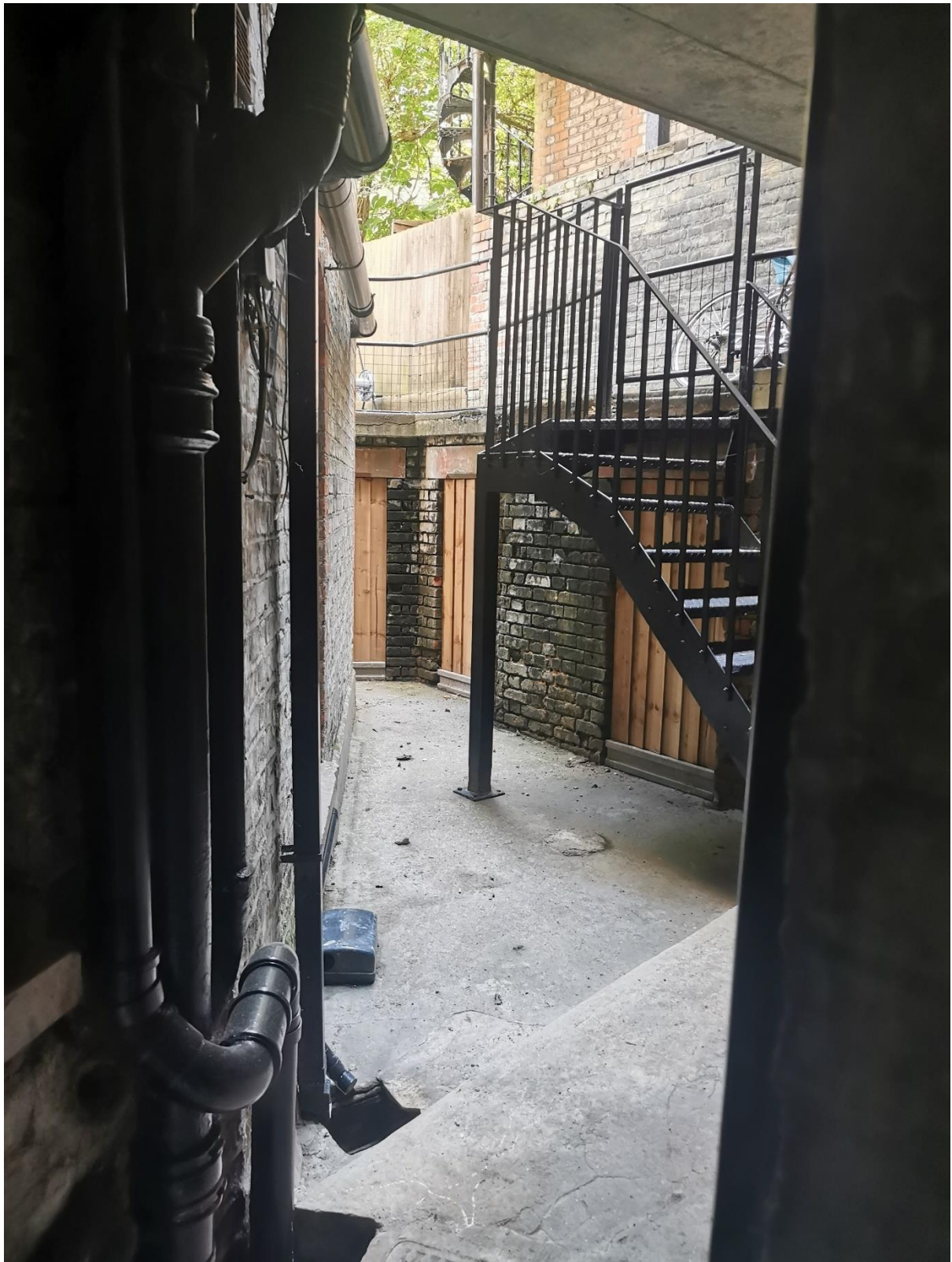
Photo 7 – External means of escape staircase and light well (viewed from bedroom French doors)
