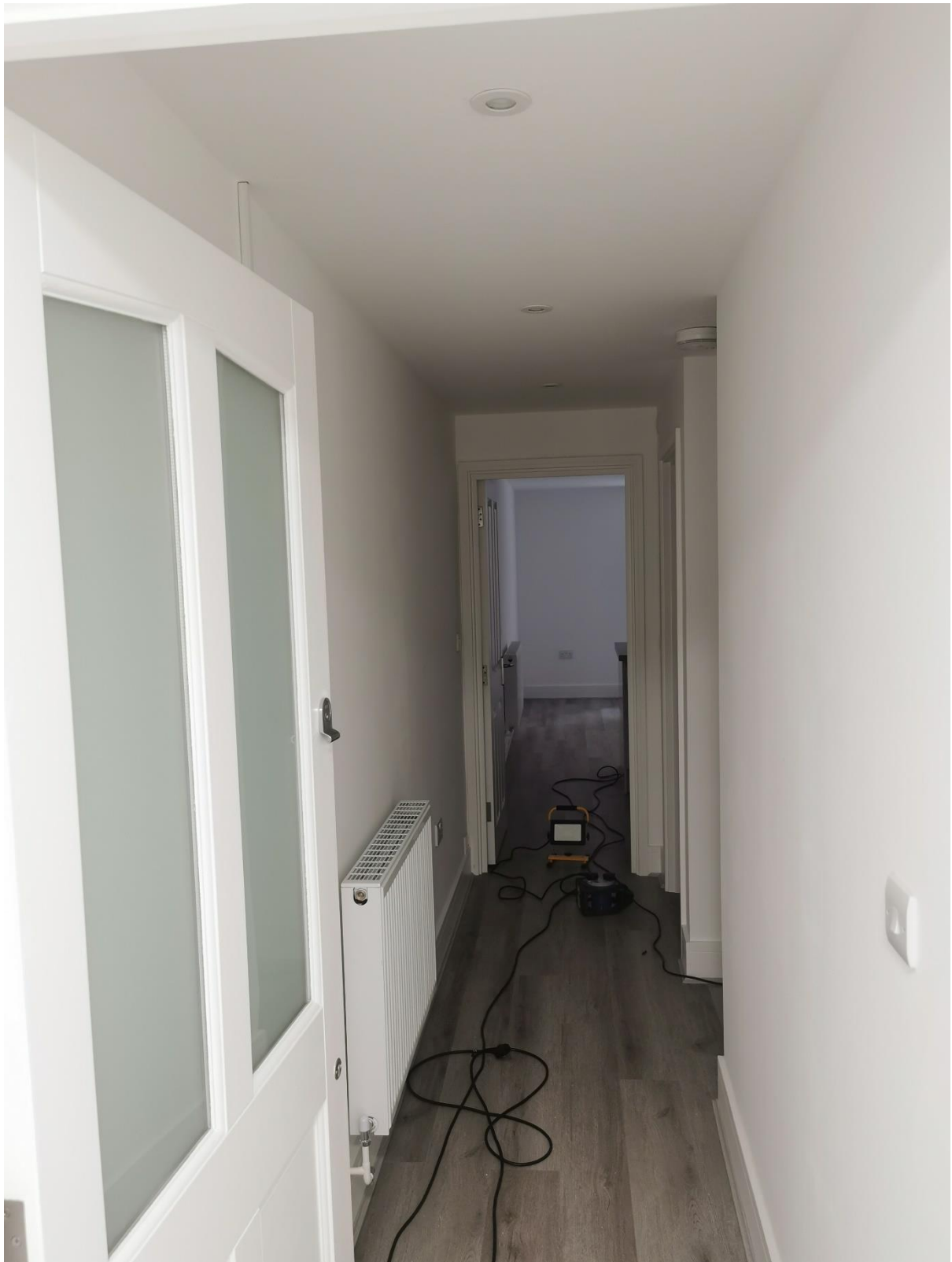
Photo 2 – Flat entrance door and internal corridor.
