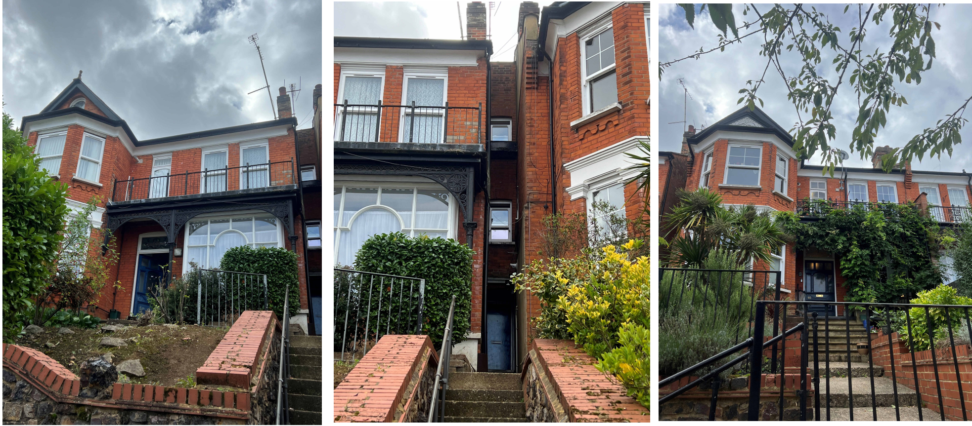
66 - 68 DUKES AVENUE FRONT ELEVATION PHOTOGRAPHS
