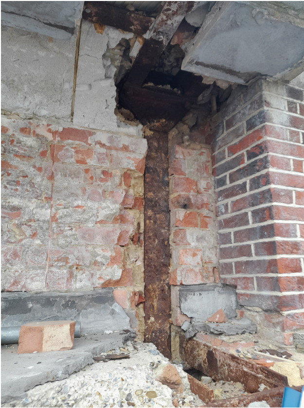
Exposed steel column at cornice level.
