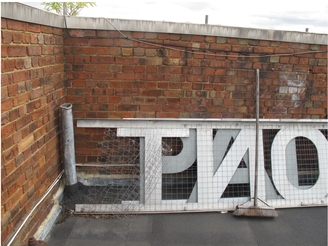
4. Rear of front elevation
