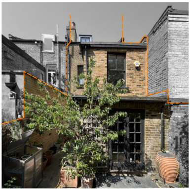
Photo: Garden elevation of 20 Townsend Road
