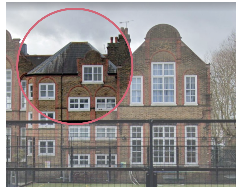
Roof form on the Campsbourne School, opposite the site
