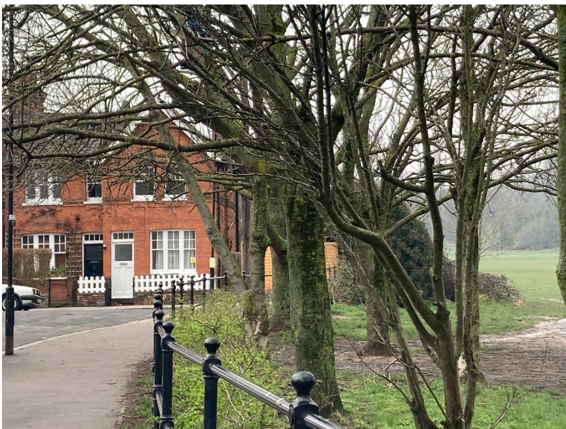
Newland Road view taken closer to No 175. Landscaping obscures views of the side garden until one is standing very close to it. The park rail is modern.
