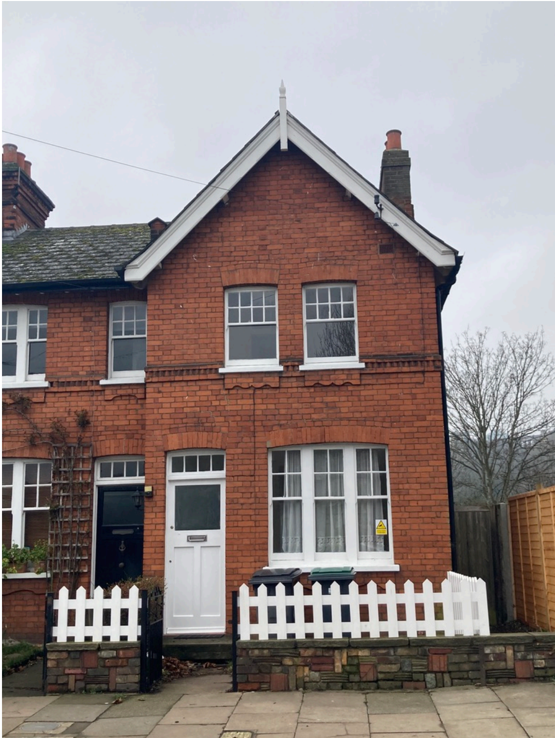
The front elevation to Nightingale Lane. The fencing and dwarf wall are modern.
