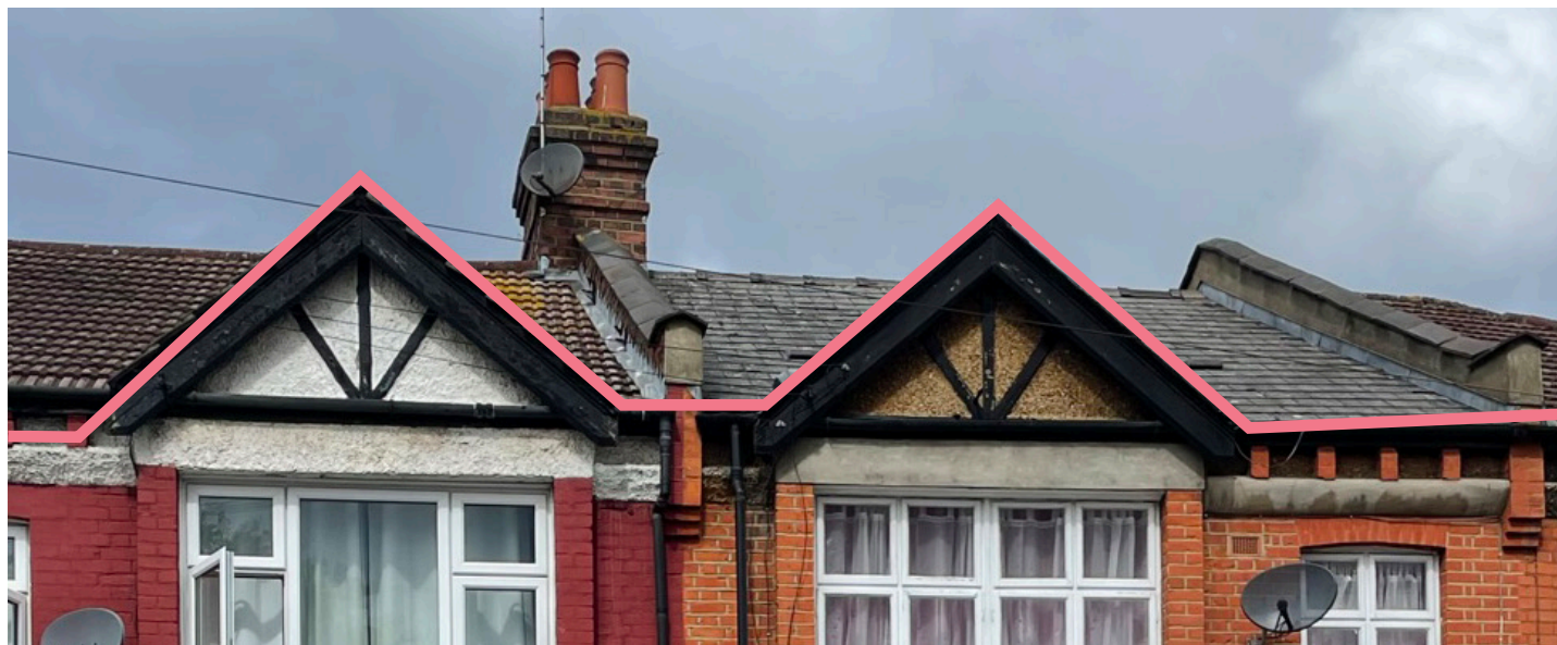
Roof form - No.91-99 Nightingale Lane
