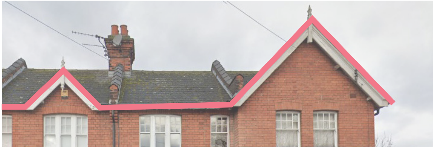
Roof form - No.171-175 Nightingale Lane
