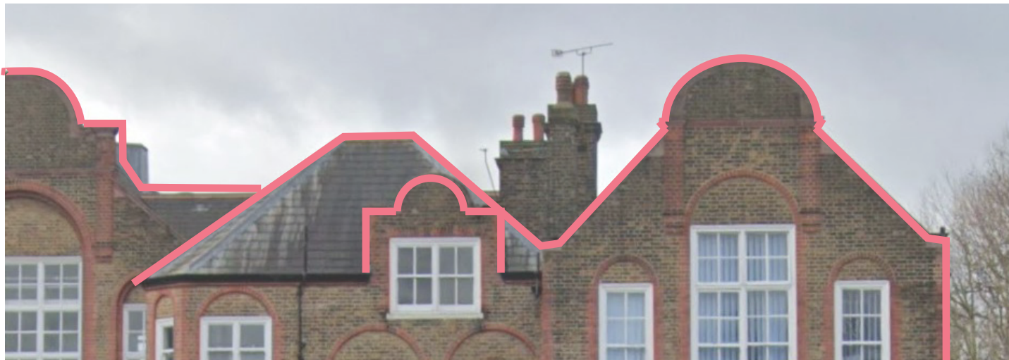
Roof form - Campsbourne School
