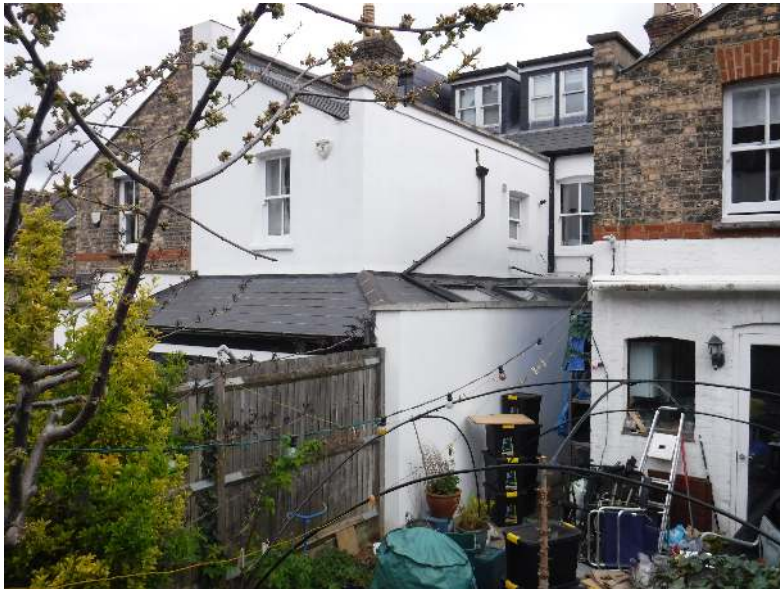
Rear elevation showing extension to no. 4 beyond
