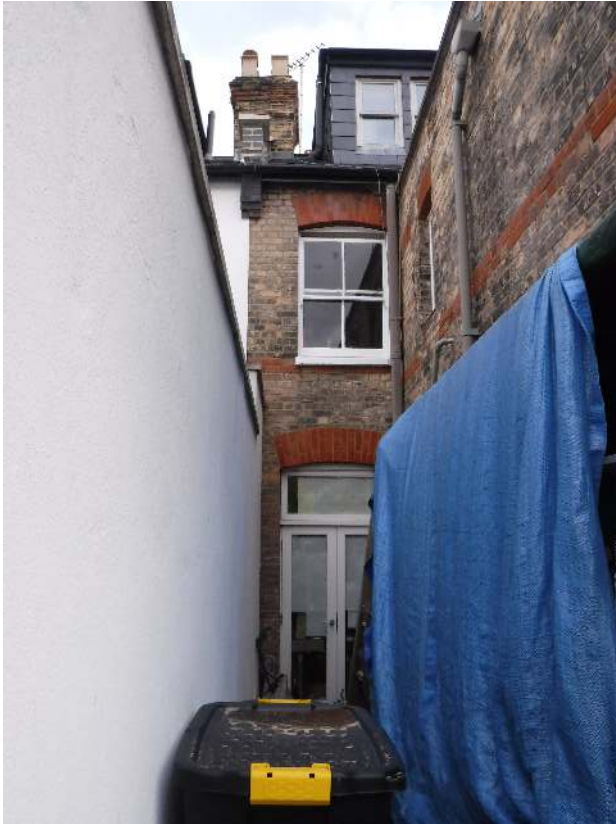
View of side passage, showing flank wall of similar extension to 4 Bryanstone Road
