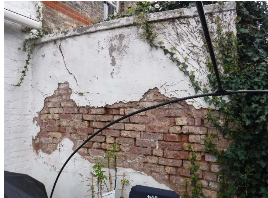
View of boundary wall with 8 Bryanstone Road to be rebuilt to form flank wall of proposed extension
