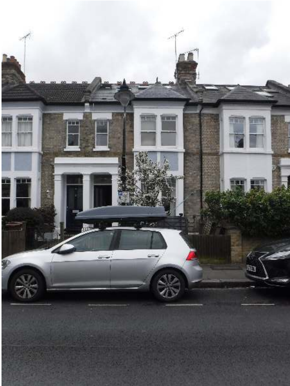
Front elevation: general view
