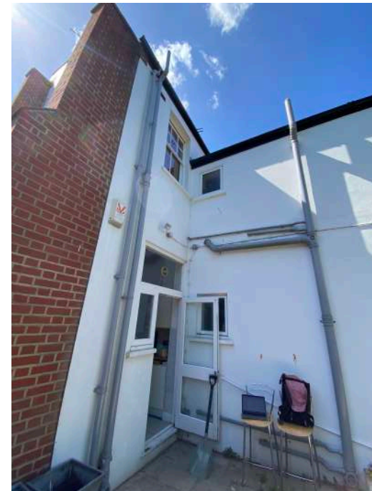
Rear Elevation (taken from GF flat rear garden upper level which will become the extension)
