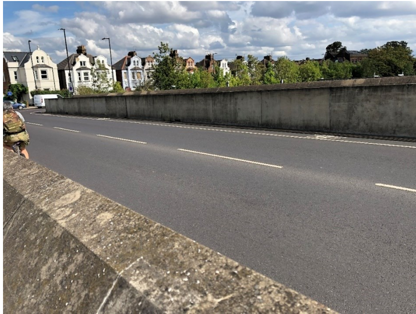
Photograph 4.7: Cycle lanes along Buckingham Road Bridge
