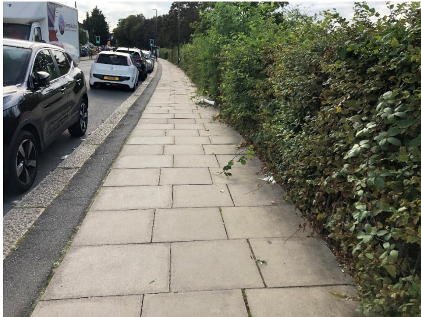
Photograph 4.3: Footway along the northern side of Albert Road
