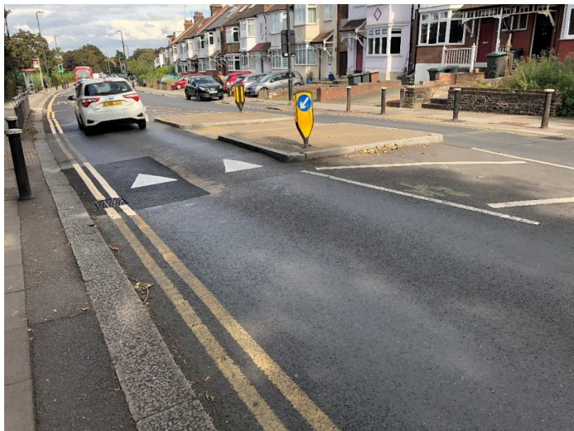
Photograph 4.2: Pedestrian refuge island crossing between Victoria Road bus stops along Albert Road
