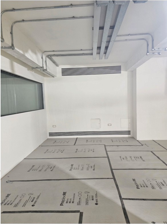
Where FCU are behind new wall linings such as in the supper room with no previous grilles to reference - modern plastered in slot grilles have been installed.
