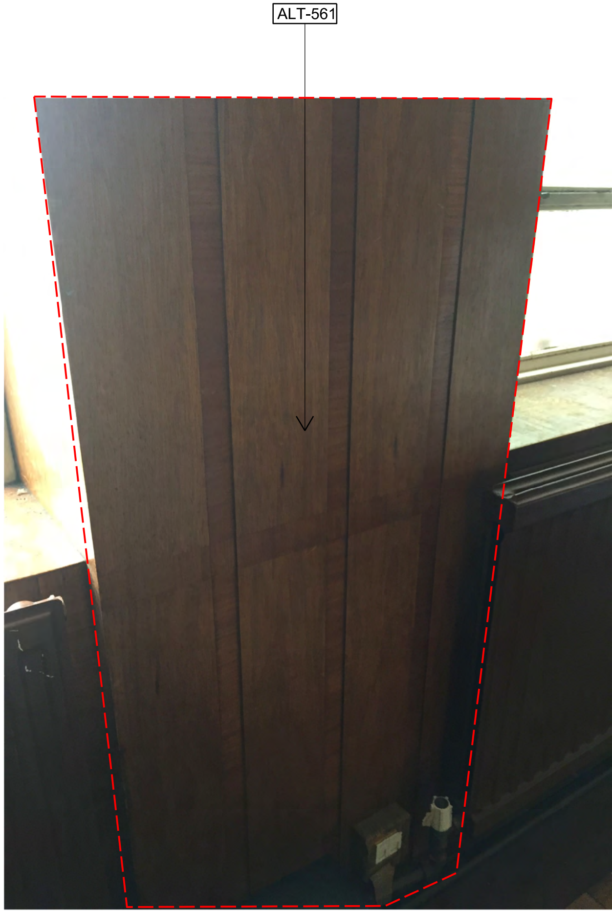
05 Existing timber wall lining 1:NTS
