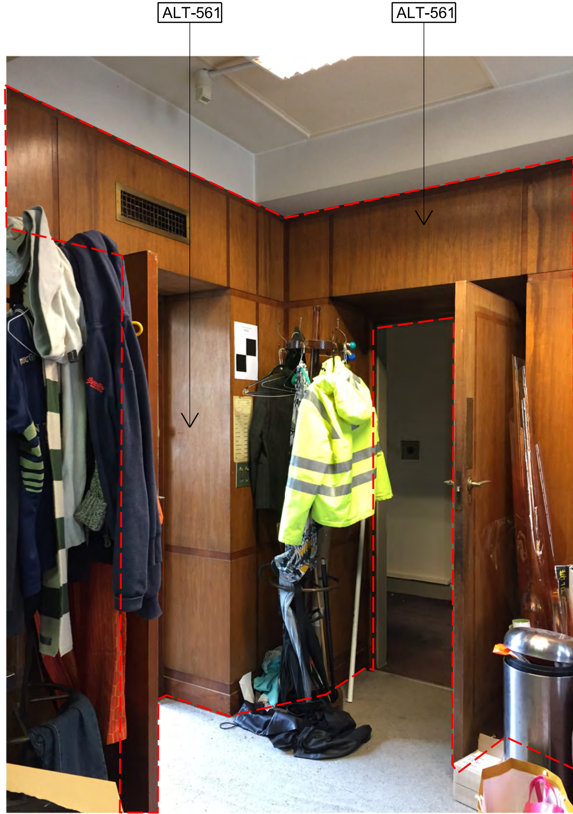
06 Existing timber wall lining 1:NTS
