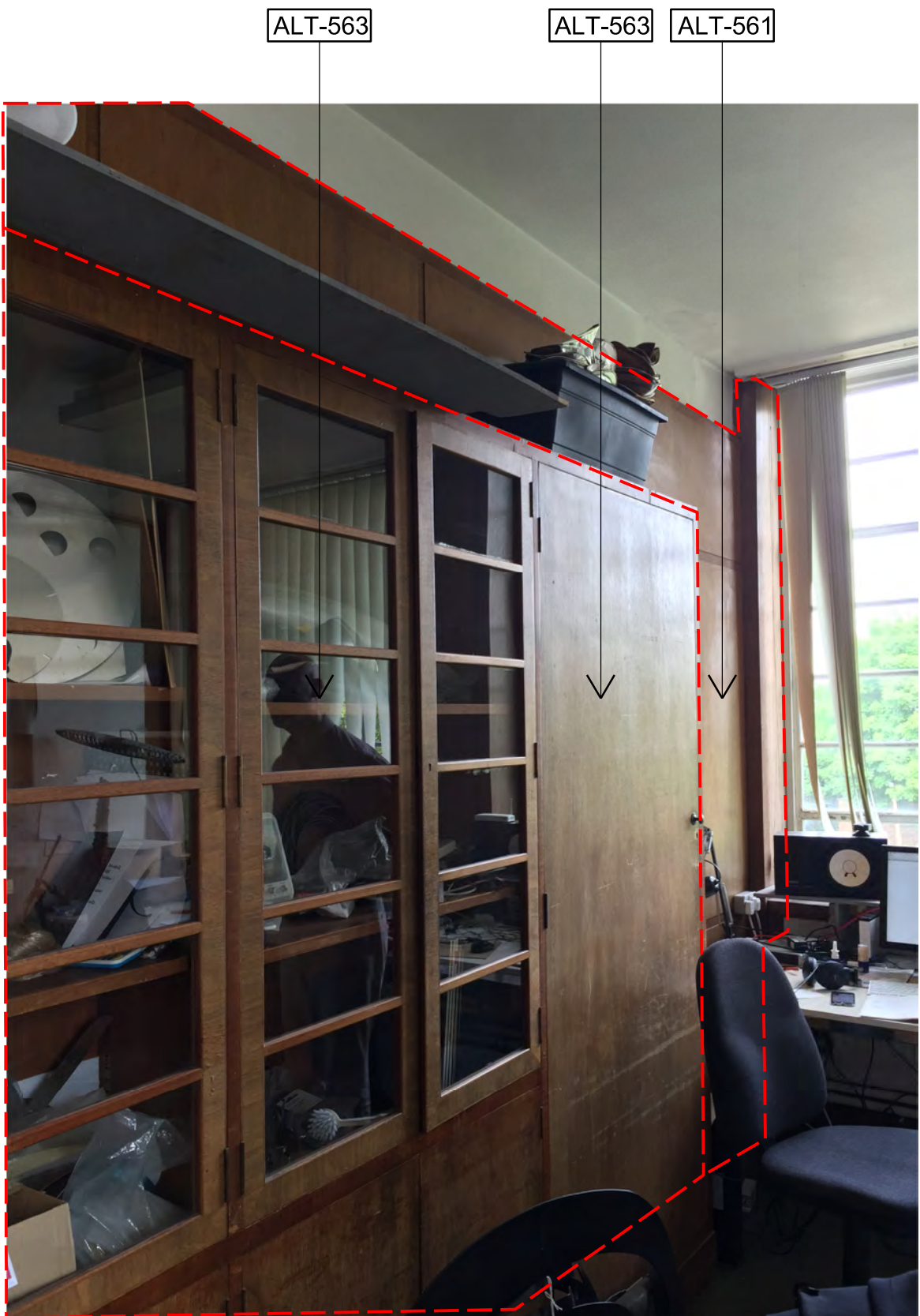
02 Existing joinery & timber wall lining 1:NTS
