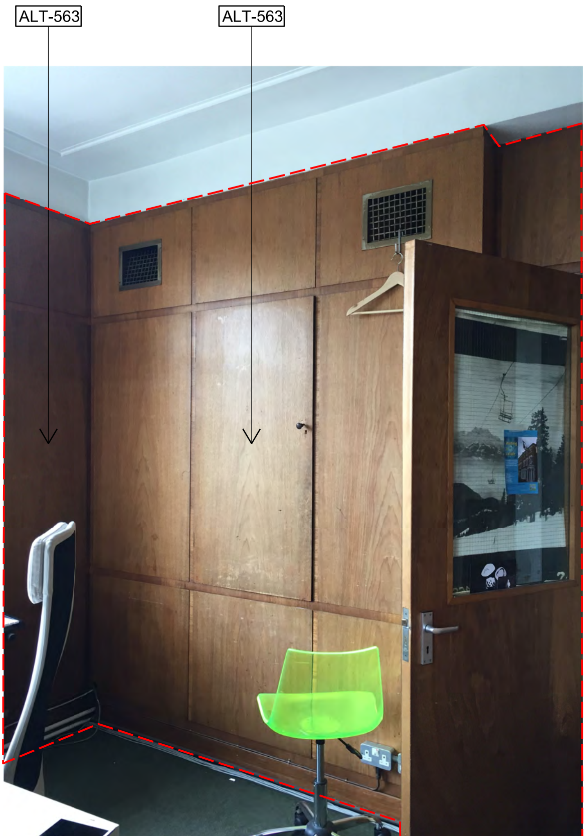
03 Existing timber wall lining 1:NTS
