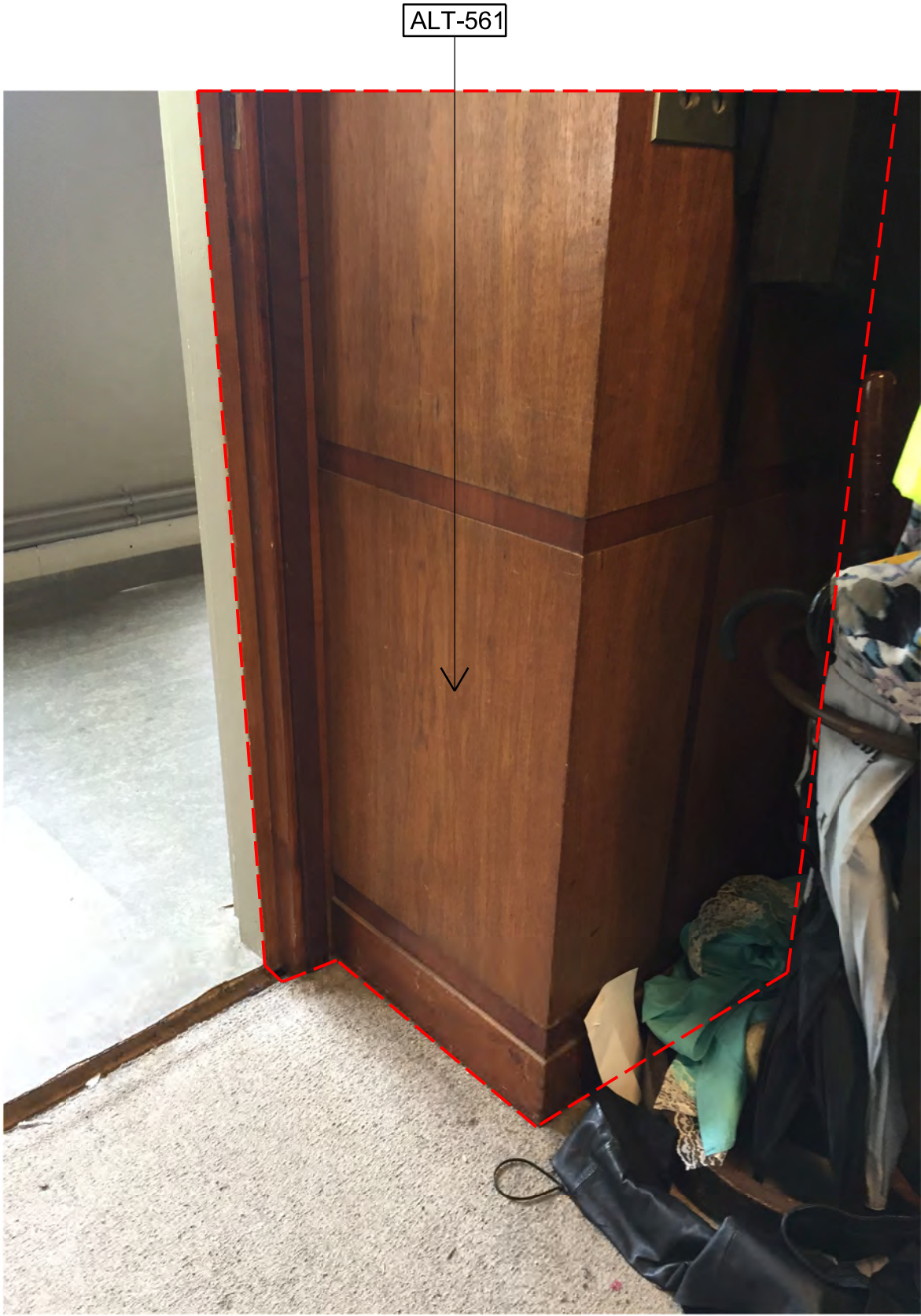
05 Existing timber wall lining 1:NTS
