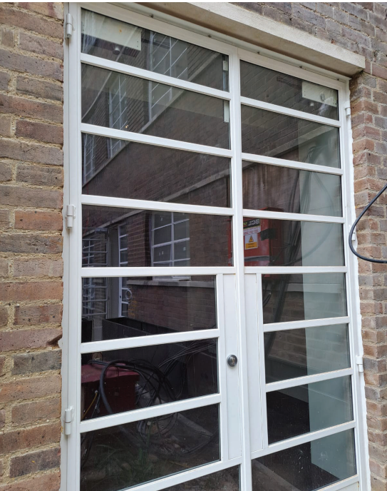
New crittall window/door with matching finish to refurbished windows.
