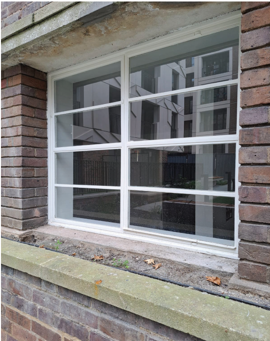
Typical existing refurbished crittall window white paint finish.
