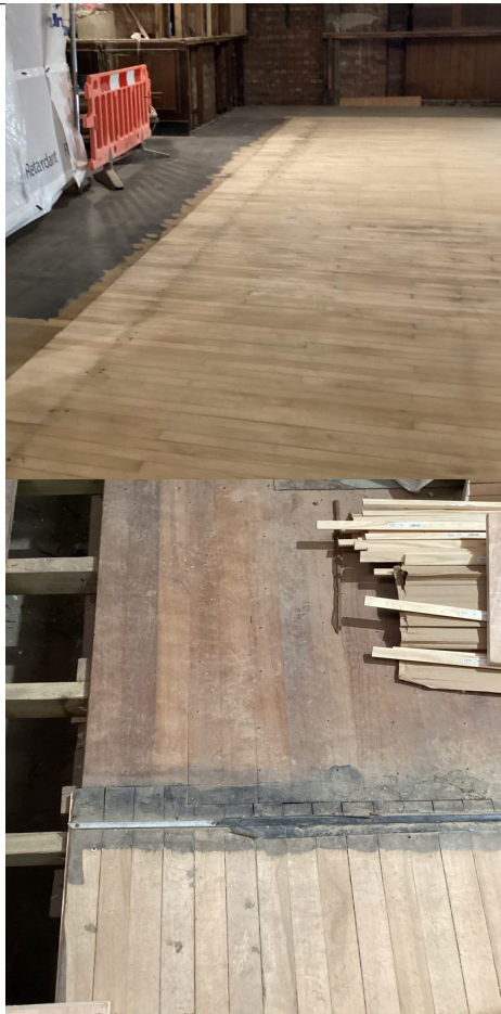
Assembly Hall Original floor stained and marked, flooring to be repaired as method statement ALT-531
