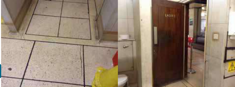
Lavatories Terrazzo floors run into the lavatories, similar to the entrance's damage is mostly minor cracking, with scratches notable from cubicle doors. Light repairs are required as method statement ALT-411 and ALT-412
