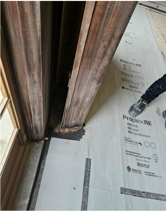
To reduce the impact on the original panelling, sockets have been installed within the original curtain recesses
