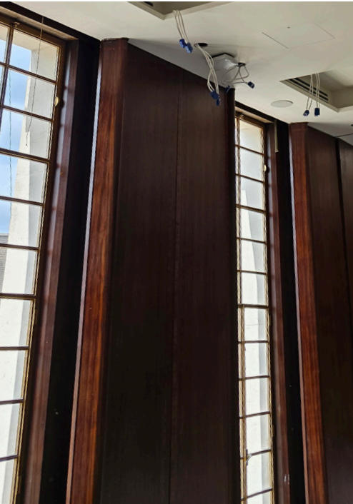
ALT-559 Refurbishment of veneered wall lining The existing walnut veneered panelling was in a general condition and it to be refurbished to a near new condition. An approved sample of repair has been review and agreed on site and a detailed method statement of the works as the approved sample has been submitted.
