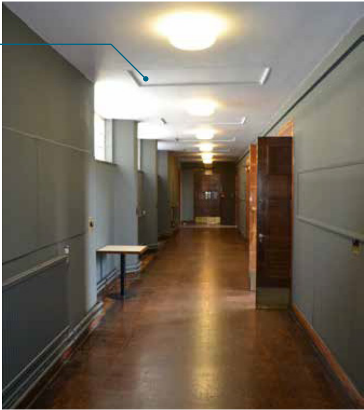
Existing radiant panels in ceiling to be removed to allow the instillation of services. To be reformed in plasterboard as insets to provide a reference to the original installation with matching trim. Original radiant panels maintained elsewhere in the building.
