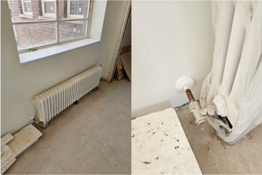
Modern existing radiators to be removed and replaced with new radiators consistently used throughout rest of existing building.
