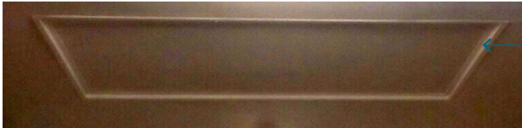
Existing radiant panels in ceiling to be removed to allow the instillation of services. To be reformed in plasterboard as insets to provide a reference to the original installation with matching trim. Original radiant panels maintained elsewhere in the building.
