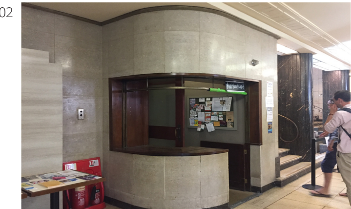
ALT 418 - Refurbishment of existing stone work
