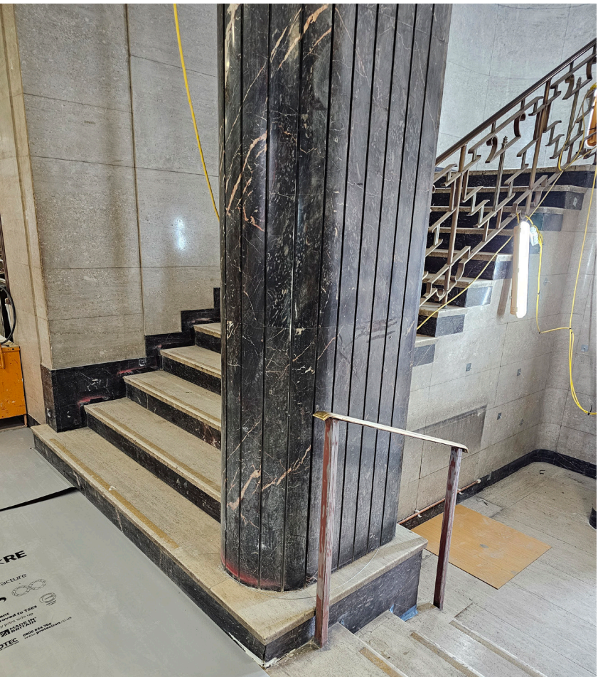
Ashburton Marble is used in feature columns and across the skirting line, it is in good condition, any loose tiles are to be re-bedded, small cracks are to be filled with a matching resin with hairline cracks and general wear maintained.
