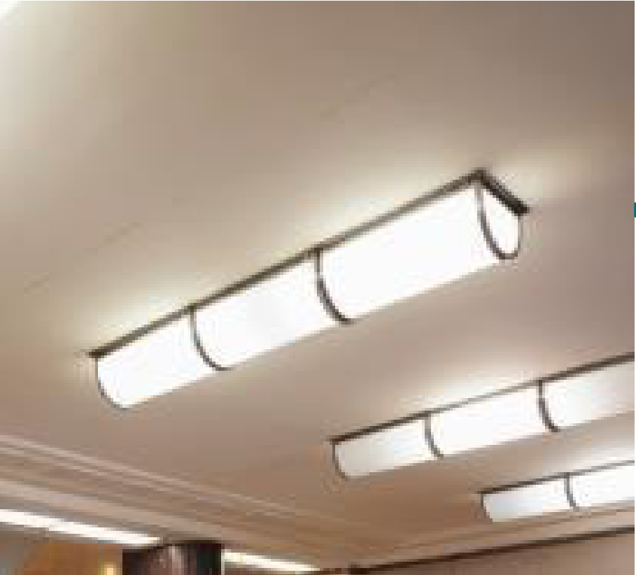
Existing half barrel strip lights X4, 345 radius, 1607 in length are to be relamped and refurbished and restored to original positions.
