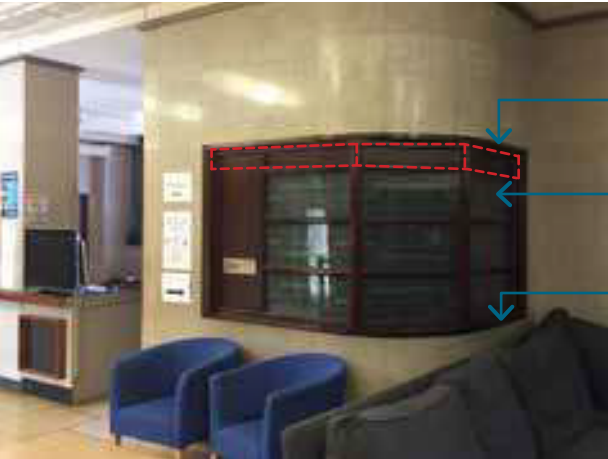
ALT-563 - Re-purposing of Existing Joinery Existing hardwood top to be refurbished, with metal frame to be replicated with new LED strip lighting as barrista room and non-original screen to be removed. With new joinery fitted below existing top and behind. As submitted drawing A5319
