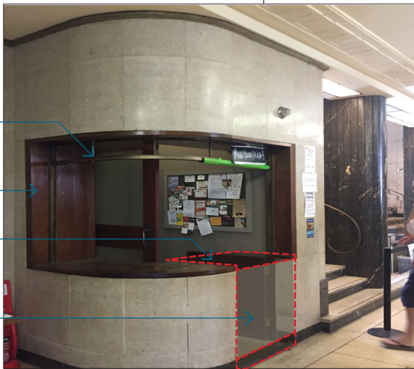
ALT-563 - Re-purposing of Existing Joinery Existing joinery to be refurbished and re-purposed as a barrista room. The existing metal frame is to be replicated with new LED trims, with existing timber top refurbished and a refill of the opening with matching stone work. As submitted drawing A5381
