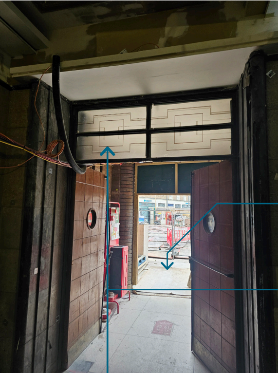
Existing skylight retained and refurbished New air-curtain above door in-front of skylight
