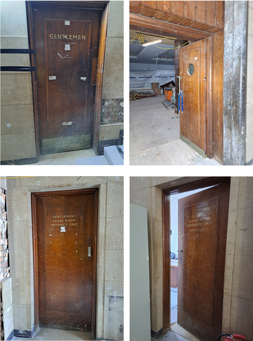
Internal Doors All the original internal doors have been retained and are to be refurbished as the relevant method statement ALT-573
