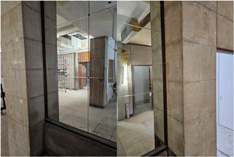
Entrance Hall Mirrors Existing mirrors with banquette seating below and bronze trims - in general good condition to be refurbished as method statement ALT-785 for mirrored wall and ALT-564 for seating below.
