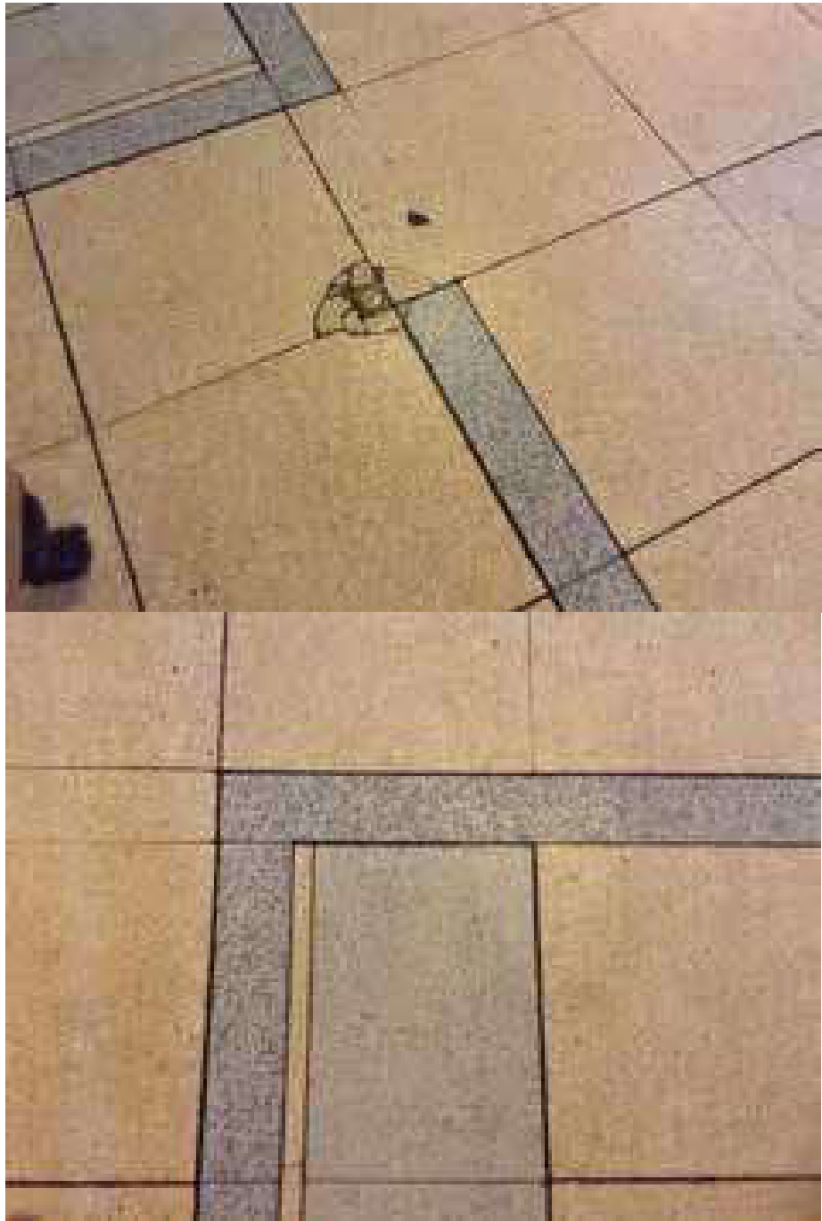
Terrazzo Floor The Foyer uses a mixture of pale blue and cream tiles. Localised areas contain mostly hairline cracks with some tiles showing larger sections of damage. The cracks are to be repaired and any tile beyond repair is to be replaced with a like-for-like finish as method statement ALT-411 and ALT-412
