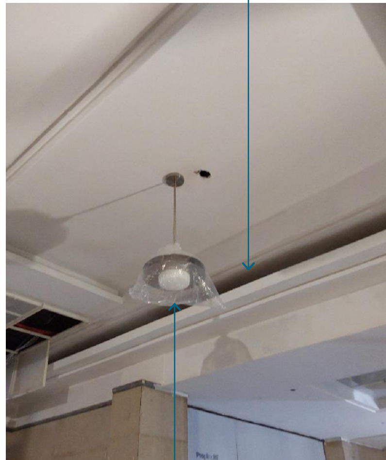
Existing pendent lights relamped, refurbished and reinstalled into existing locations
