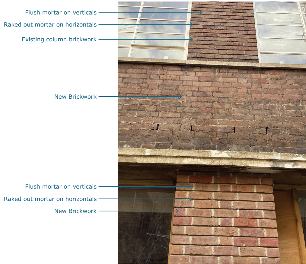
BRK-101 - The brick and bonding have been reviewed on site and approved after a previous rejection of the bricks used in block A (04/04/22), comments on approval of brick and bonding noted for the pointing to be fixed to match the existing pointing (flush on the vertical and raked out on the horizontals for columns as shown in the sample from LGF new pier) which was undertaken. Mortar is to be dyed to match the existing as the method statement for the brickwork refurbishment ALT-402.
