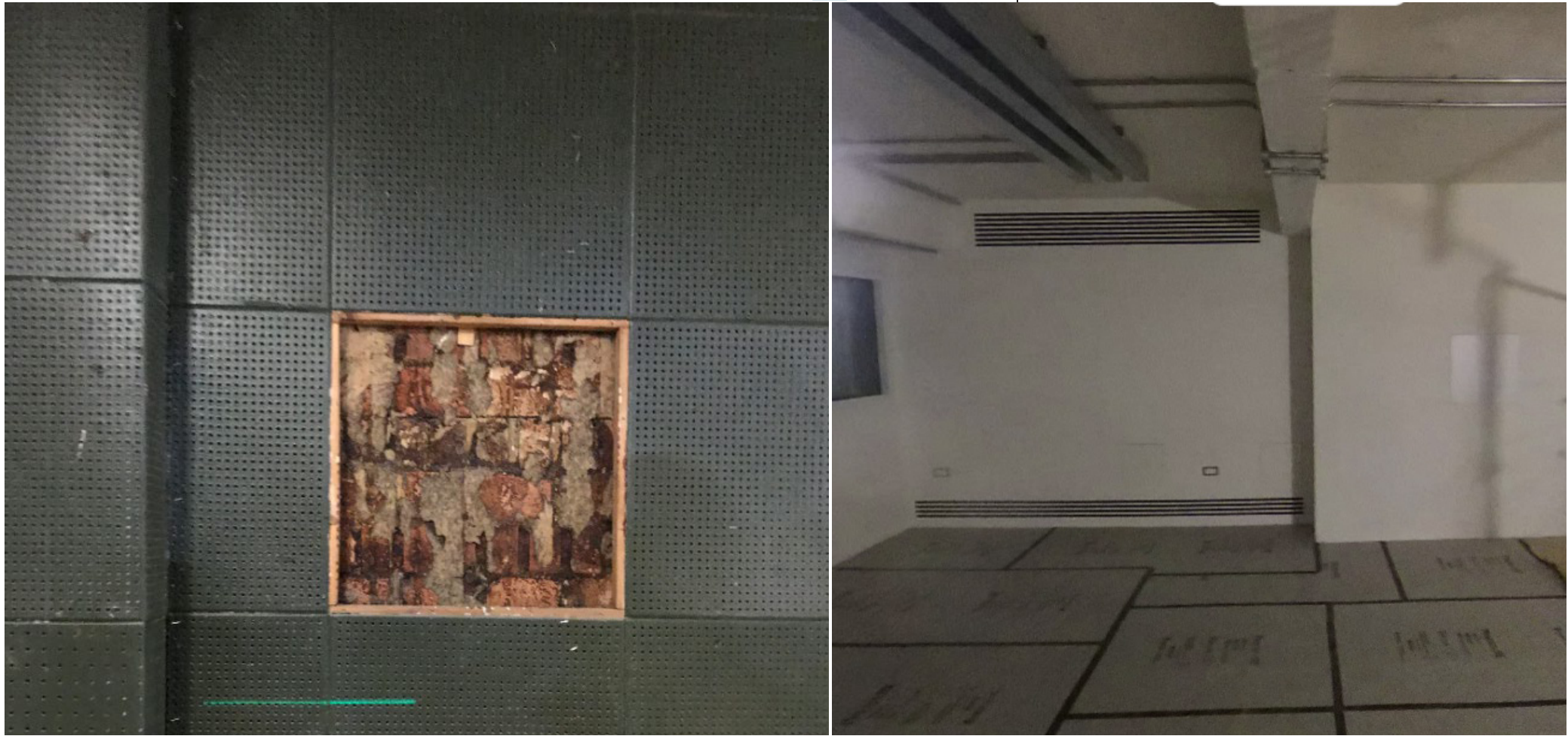
Supper Room Acoustic tiles ALT 100 - noted as having damp issues behind as well as asbestos, agreed with HE and LBH of little heritage importance and removed. New plasterboard wall with hidden services behind and plastered in ventilation grilles installed on site.
