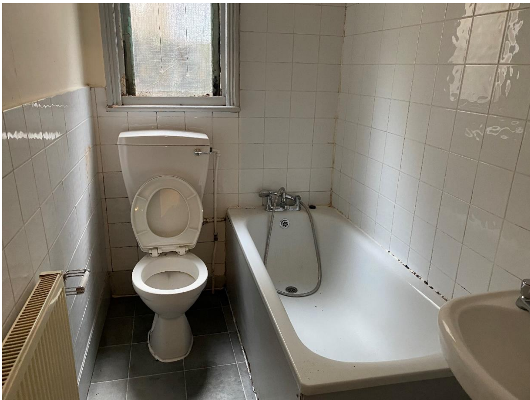
Photo 10: Bathroom in existing ground floor flat at No.3 Curzon Road
