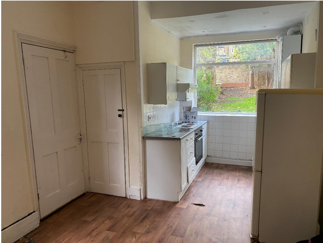
Photo 11: Kitchen in existing ground floor flat at No.3 Curzon Road
