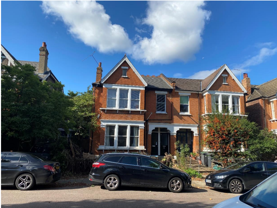
Photo 1: Frontage of Nos. 3 & 3a Curzon Road, N10, with No.5 forming 'semi-detached pair'
