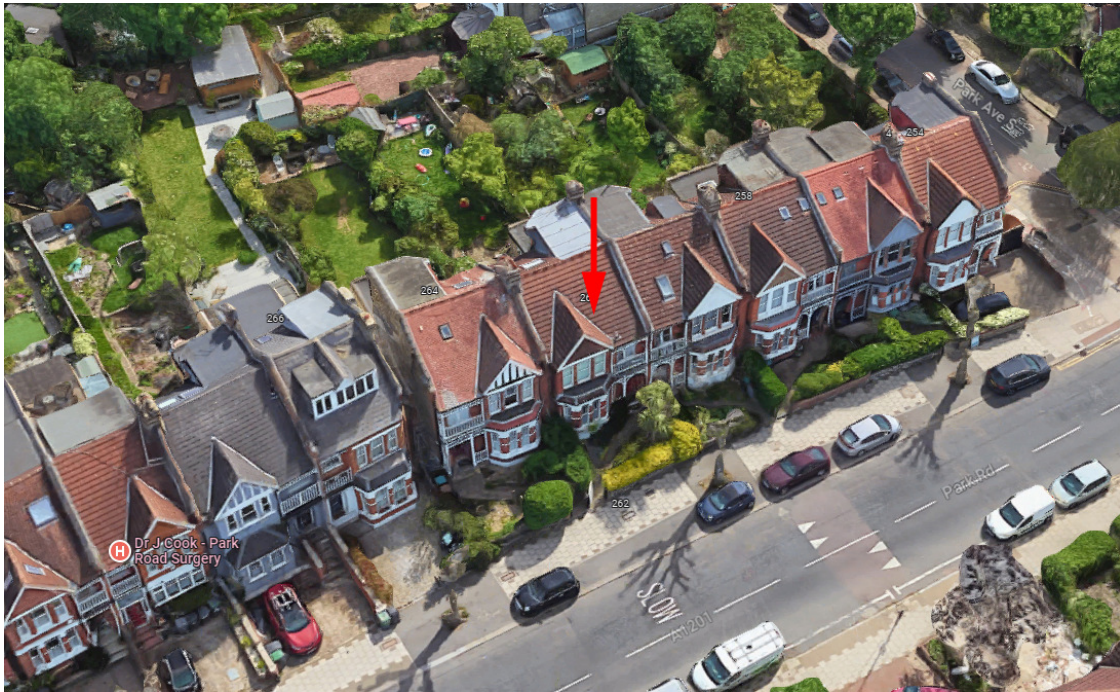
Birdseye view of the property
