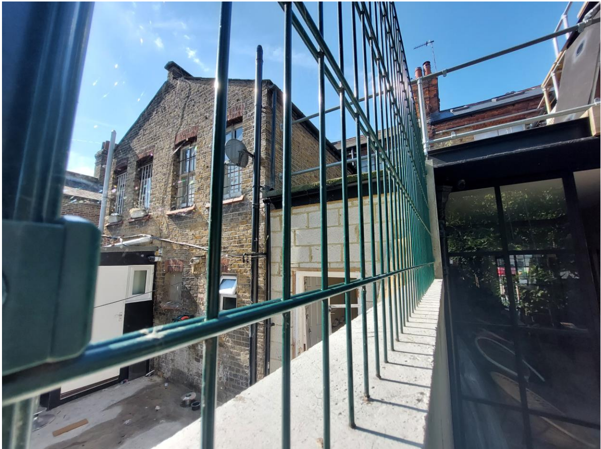
Pic.3 Rear of No.5
