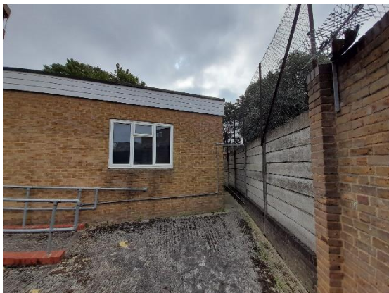
West Facing Elevation/Rear Boundary
