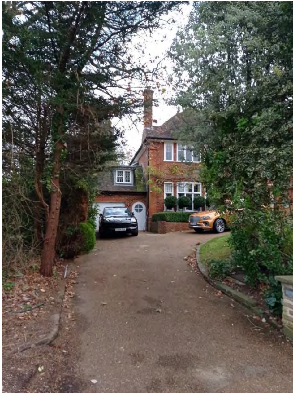
Figure 35: Brick-built garage extension to the north side of Bracken Knoll, view from the road
