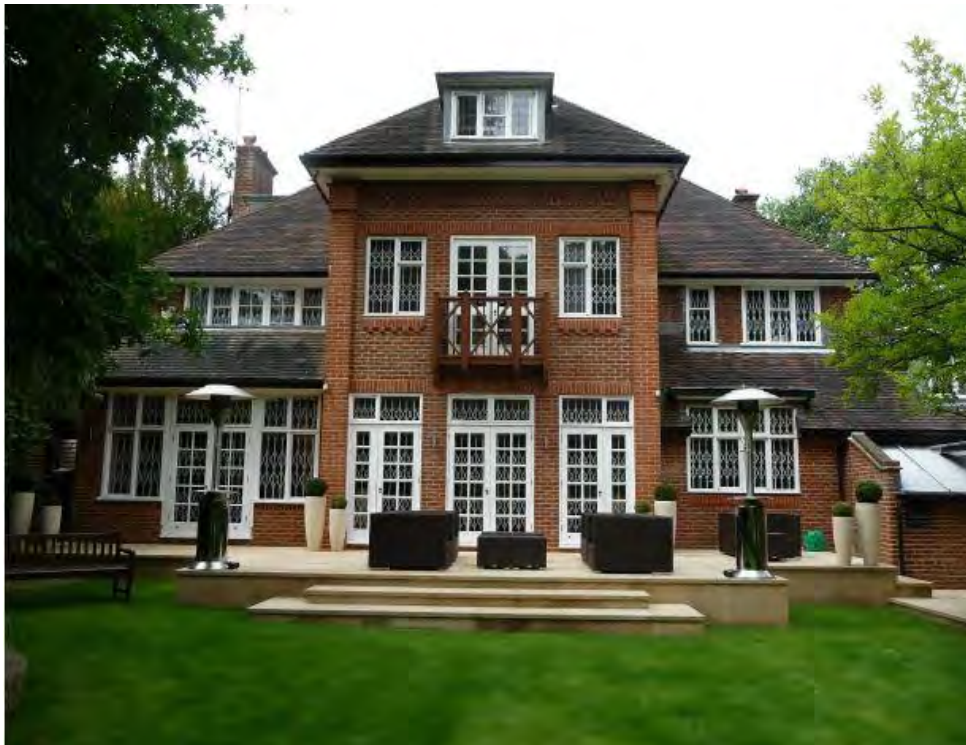
Figure 37: Rear elevation to Bracken Knoll with substantial 1990 additions; only the two windows to the first floor, right, are original to Cooper’s scheme of 1928
