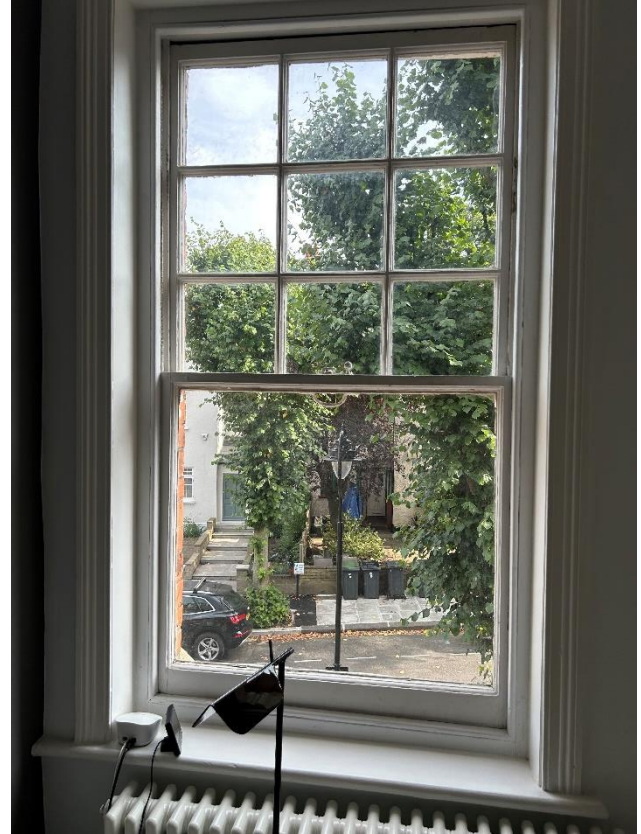
W02 Front Sash Window:
