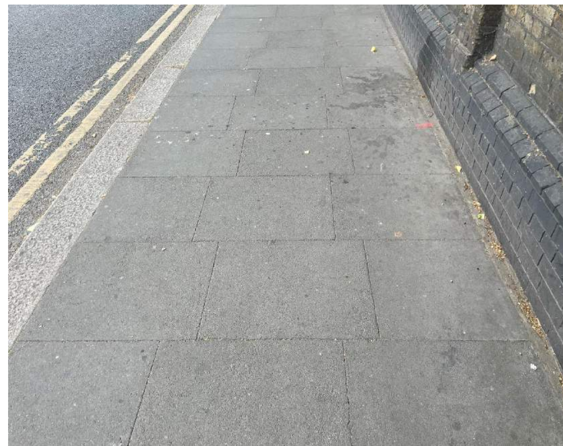
Image 27 - Parkview Rd (West) - existing wall and pavement condition
