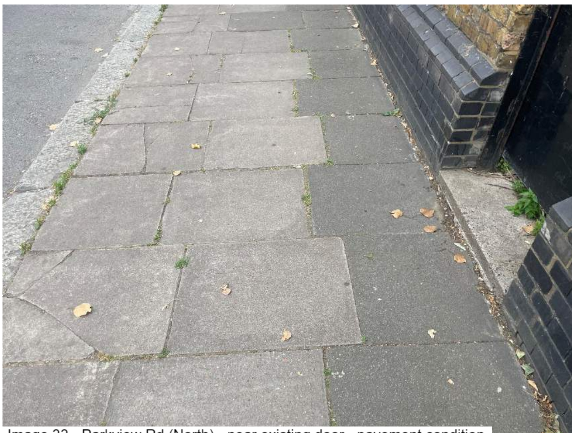
Image 33 - Parkview Rd (North) - near existing door - pavement condition
