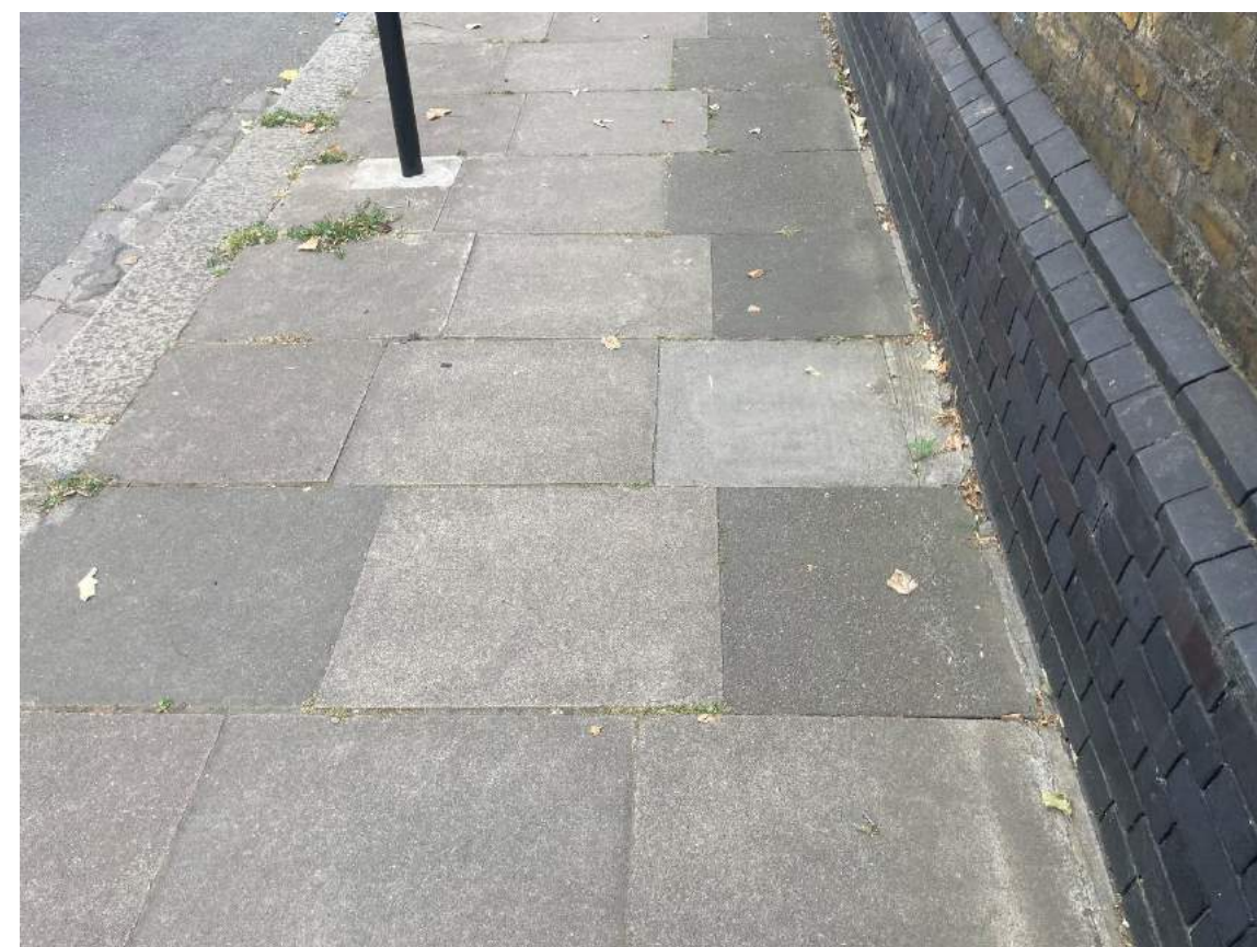
Image 36 - Parkview Rd (North) - existing pavement condition
