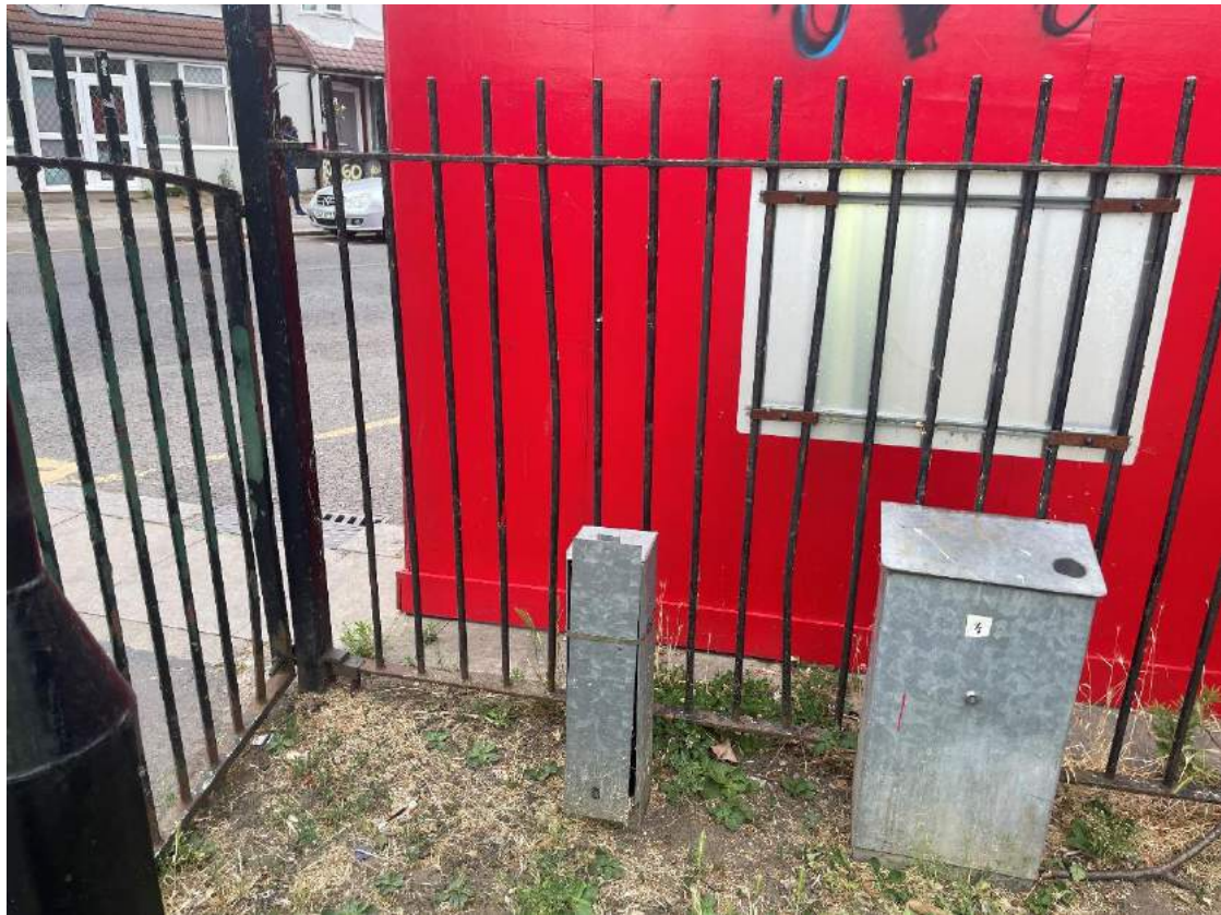
Image 10 - Parkview Rd (West) - Existing fence line, pillars & control box
