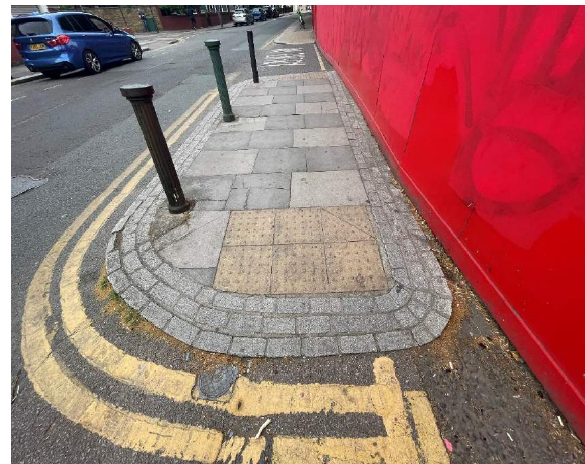
Image 15 - Parkview Rd (West) - Existing crossover
