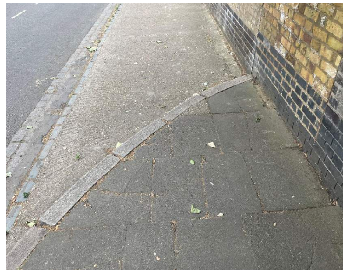
Image 54 - Parkview Rd (North) - Existing crossover
