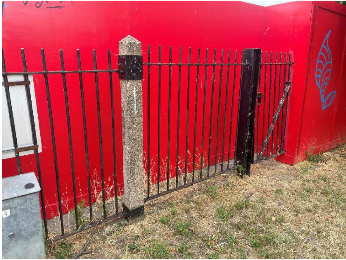
Image 9 - Parkview Rd (West) - Existing fence line and hoarding
