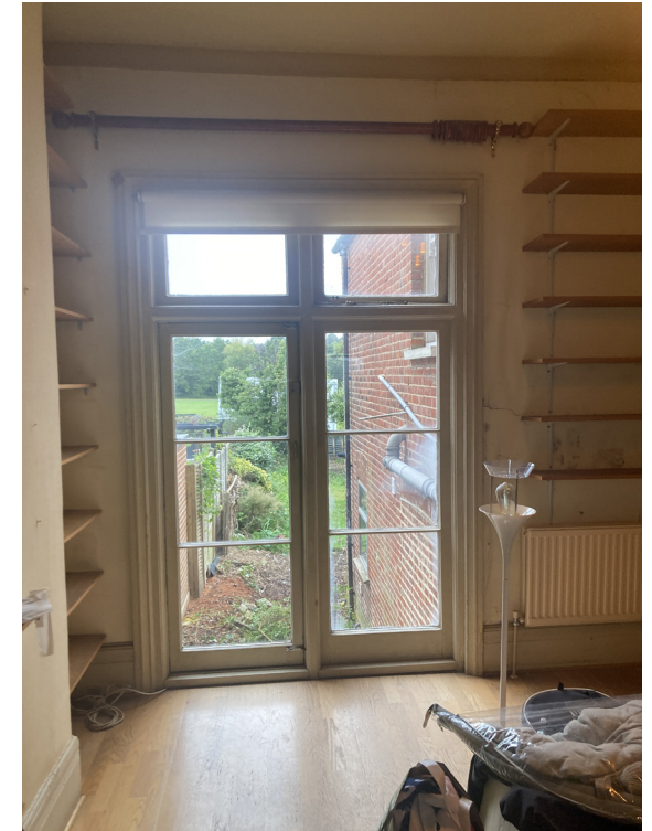
Ground floor reception looking out to rear garden
