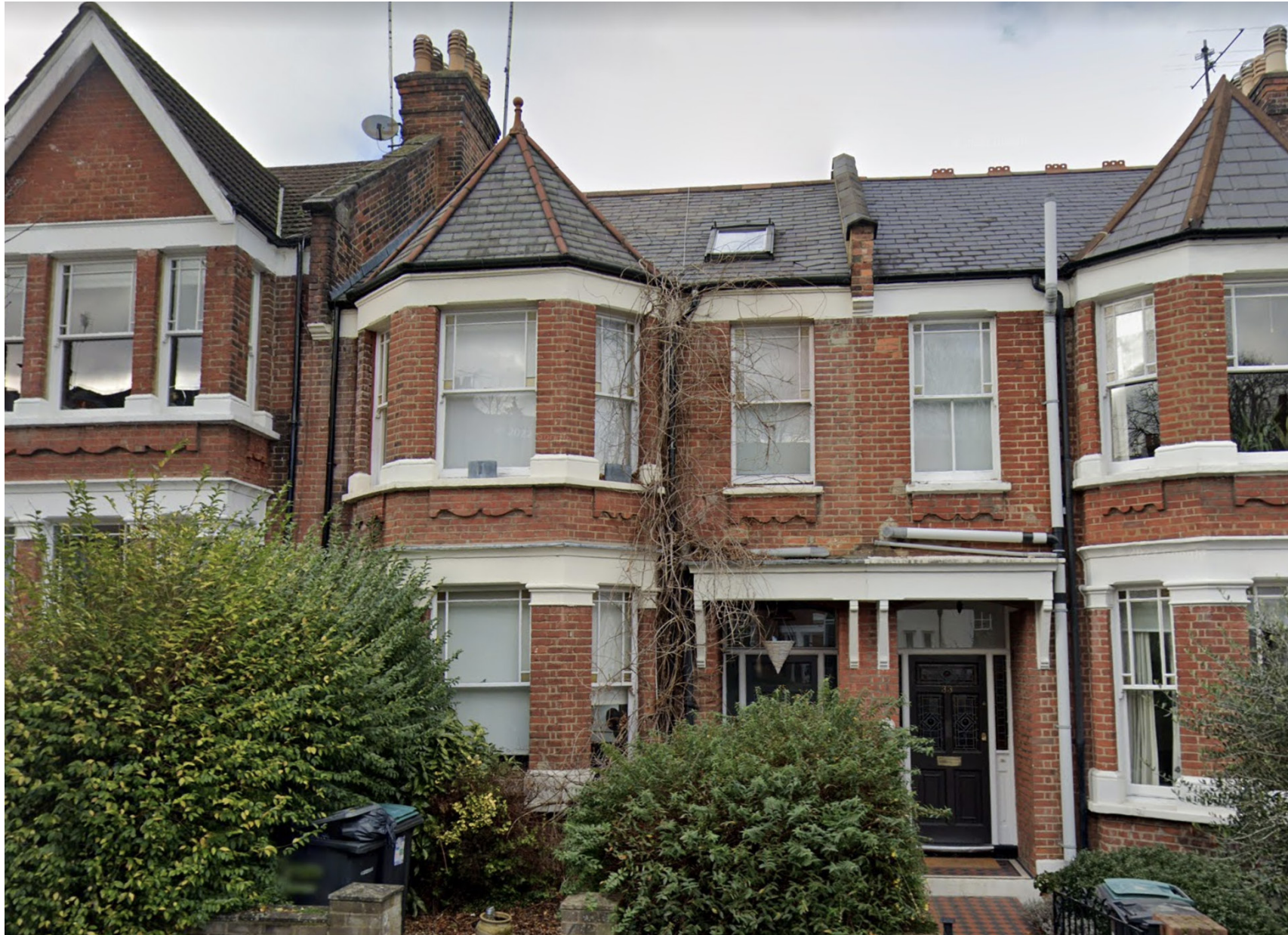
Front facade photo
