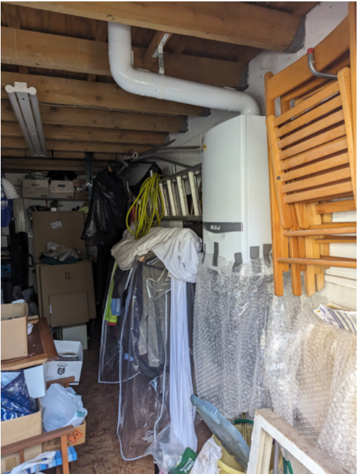
Internal View of Garage
