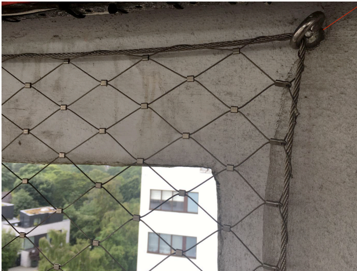
Existing opening on front block of Highpoint 1 with stainless steel Webnet guarding -fixing details to be replicated
