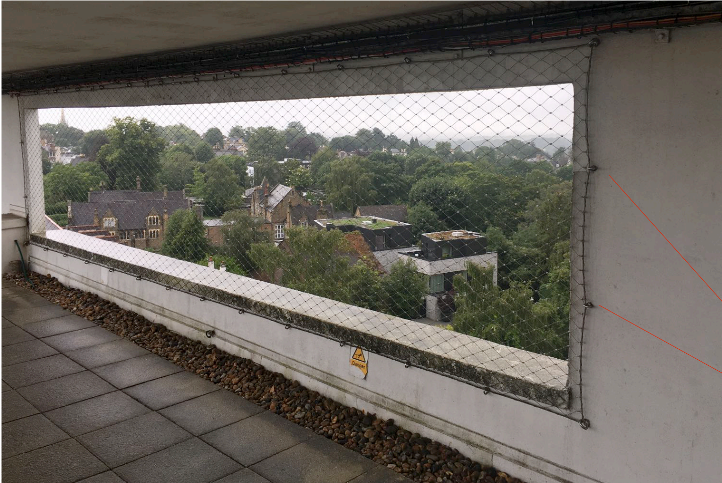
Existing opening on front block of Highpoint 1 with stainless steel Webnet guarding -fixing details to be replicated
