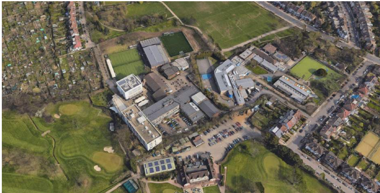
Fig 3: 3D satellite Image of the site
