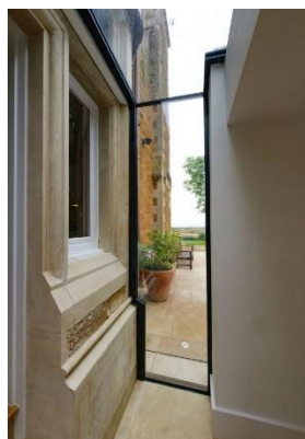
Glazed link between new and old
