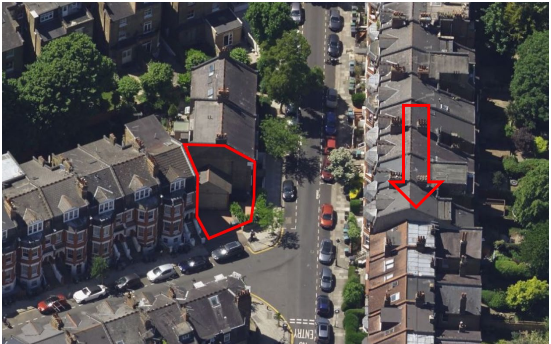
The development site at the junction of Milton Park and Milton Road.
