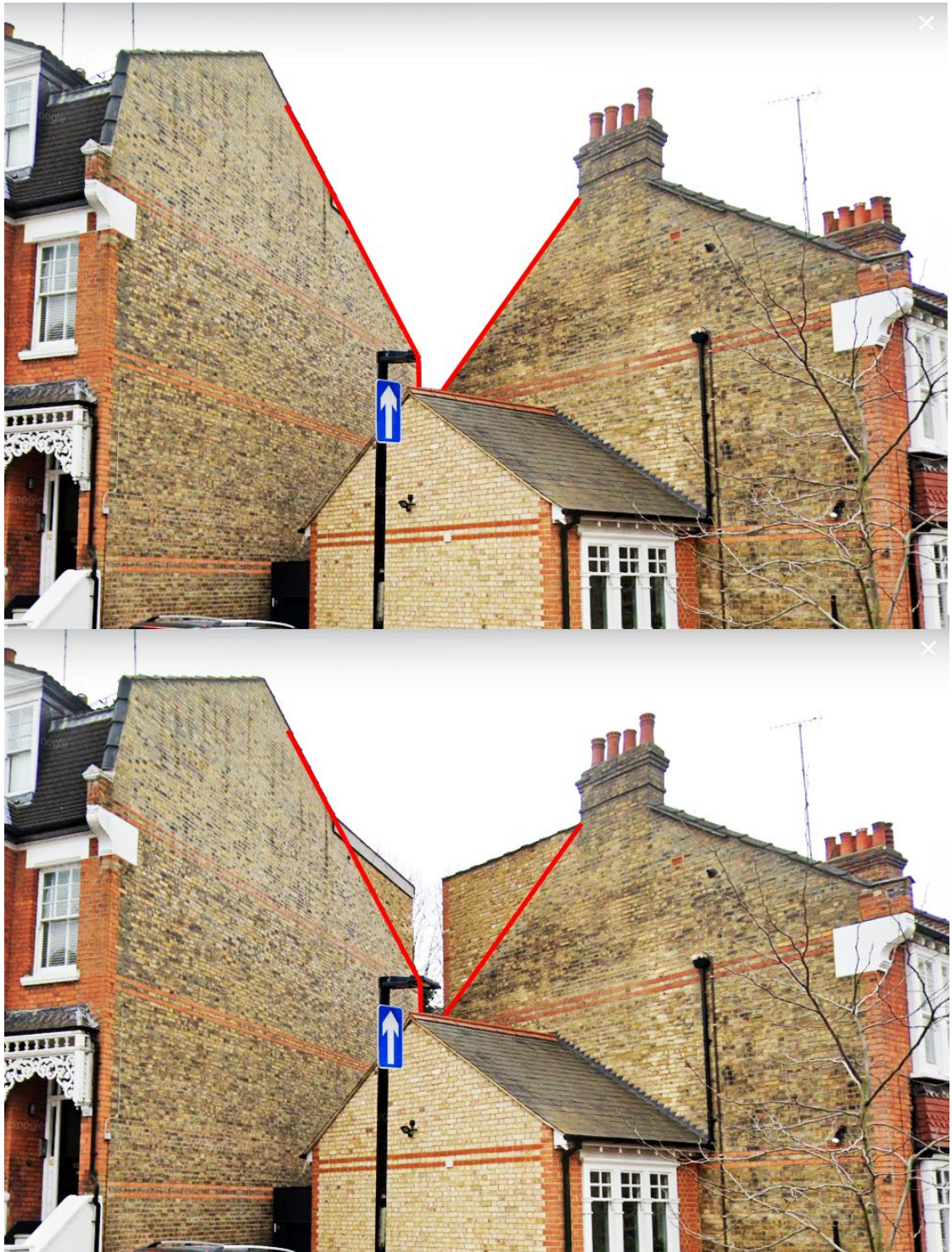
29 Milton Road (left), 29 Milton Park (right) – original roof profile above.
