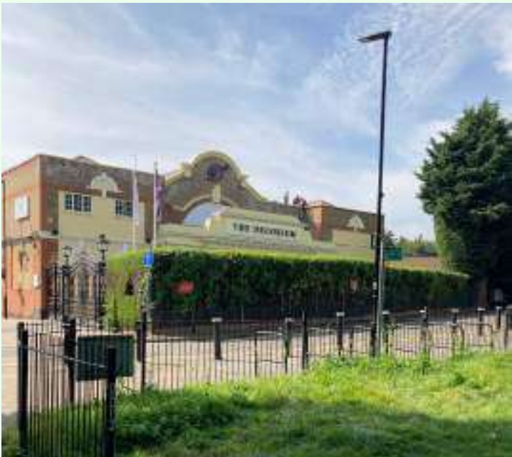
2. The Decorium - Locally listed building of merit, set behind a hedge which partially screens views from the Common.
