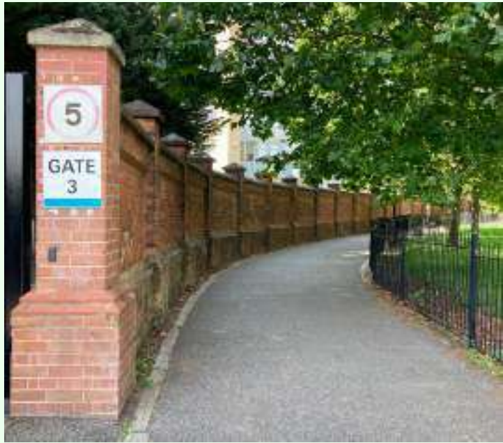
1. Wall on south side of Common - Statutory listed structure.
