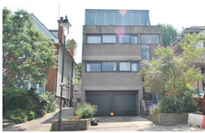
No 7 Cholmeley Crescent
