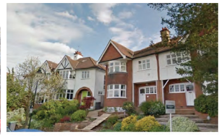
No 23-25 Cholmeley Crescent
