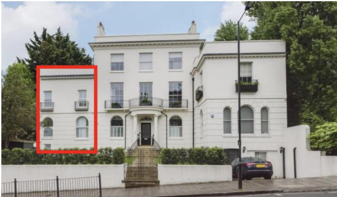
Image 1: The West façade of St George's Terrace as viewed from North Hill. 1 Park House Passage is outlined in red.
