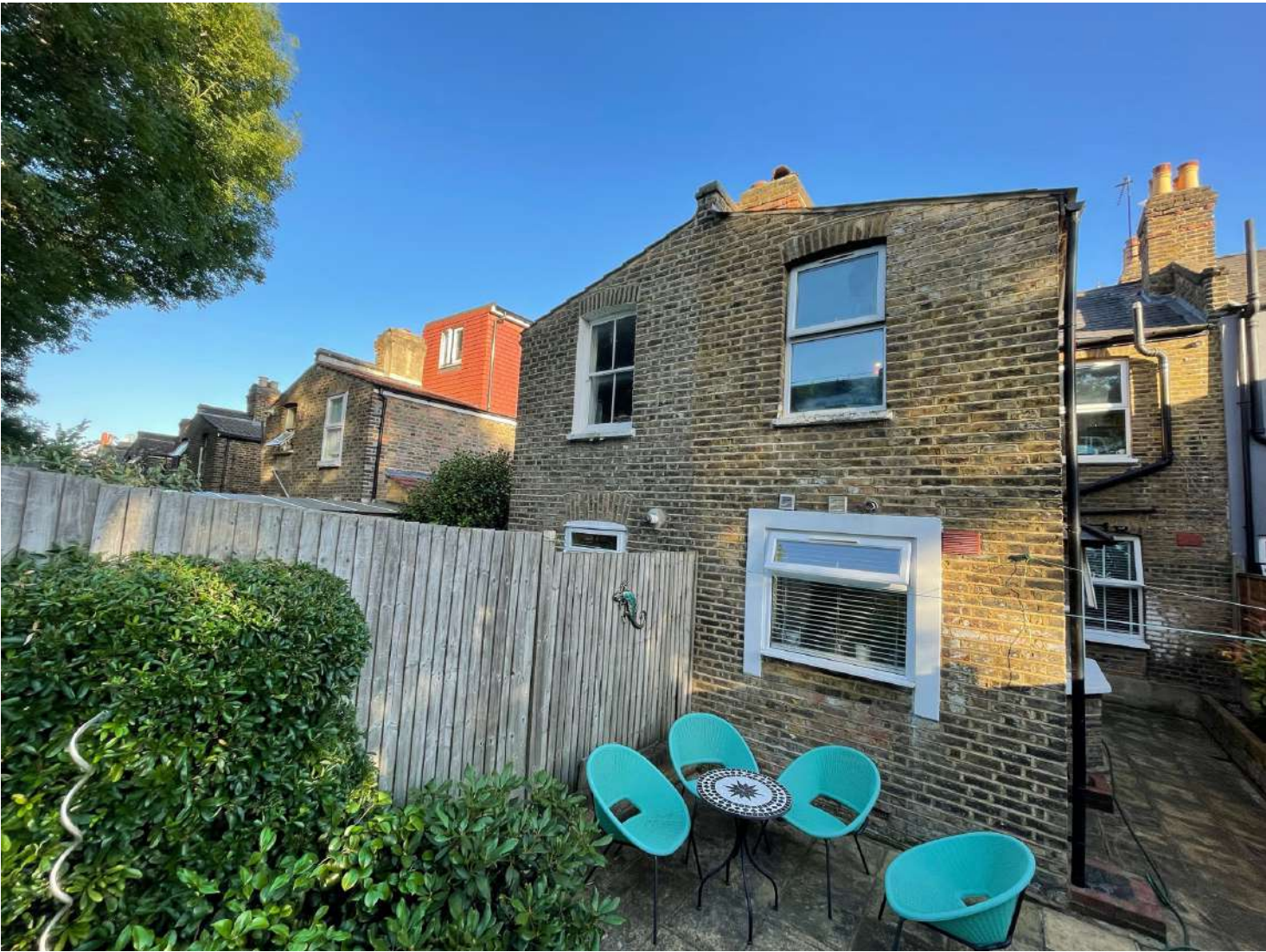
Photo taken standing in the back garden, looking to the west of the property.
