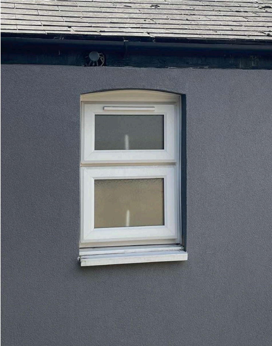
Photo of neighbour’s bathroom window (original size of 0.7m wide by 1.0m high) at 21 Cranbrook Park - first floor flat.
