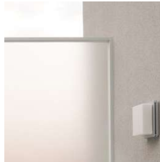
1. Translucent balustrade with aluminium handrail
