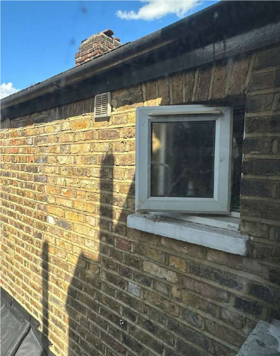
Photo of existing bathroom window at 23B Cranbrook Park, with dashed outline of where original bathroom window used to be.
