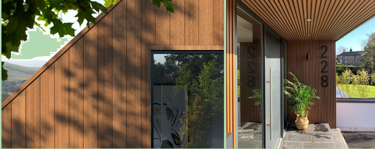
As Built examples of External Cladding
