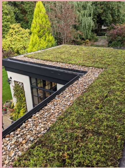
Flat Roof: Green Roof
