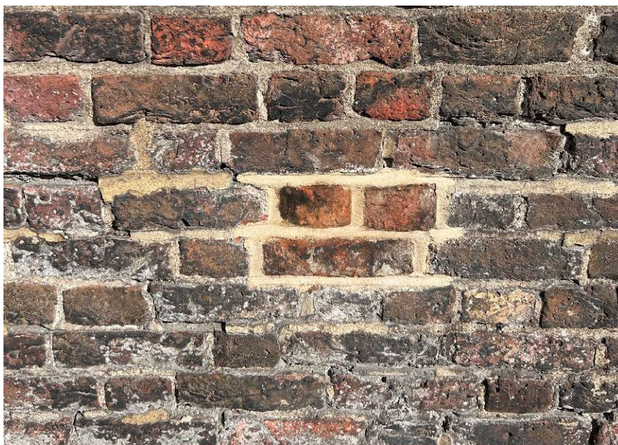
Replacement brick panel
