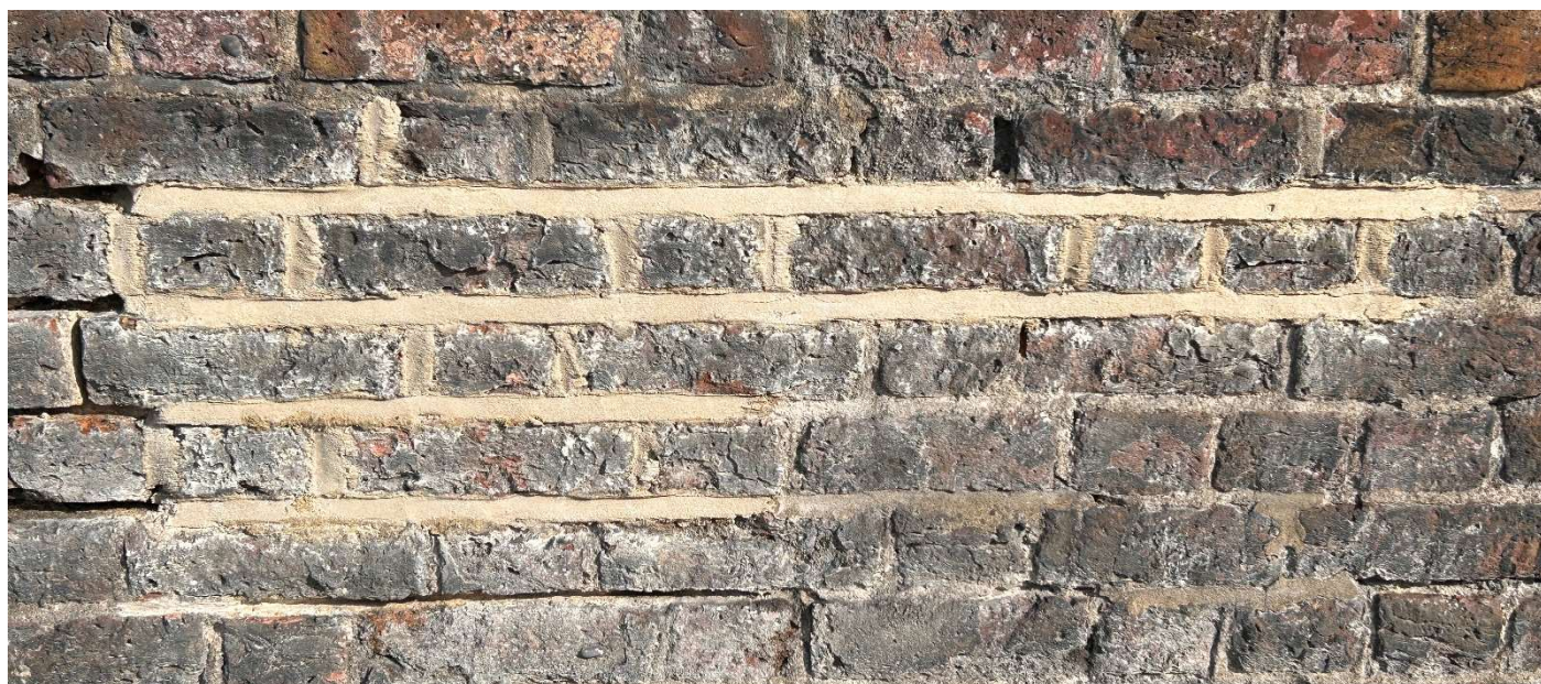
Weather struck pointing detail
