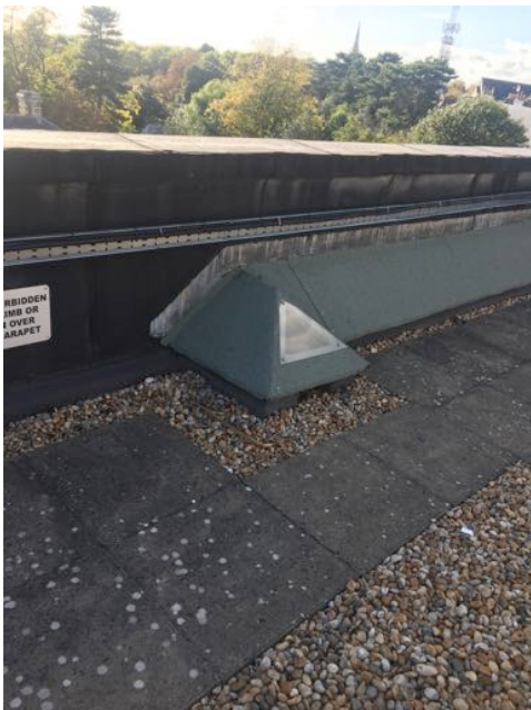
Typical conditions at the parapet
