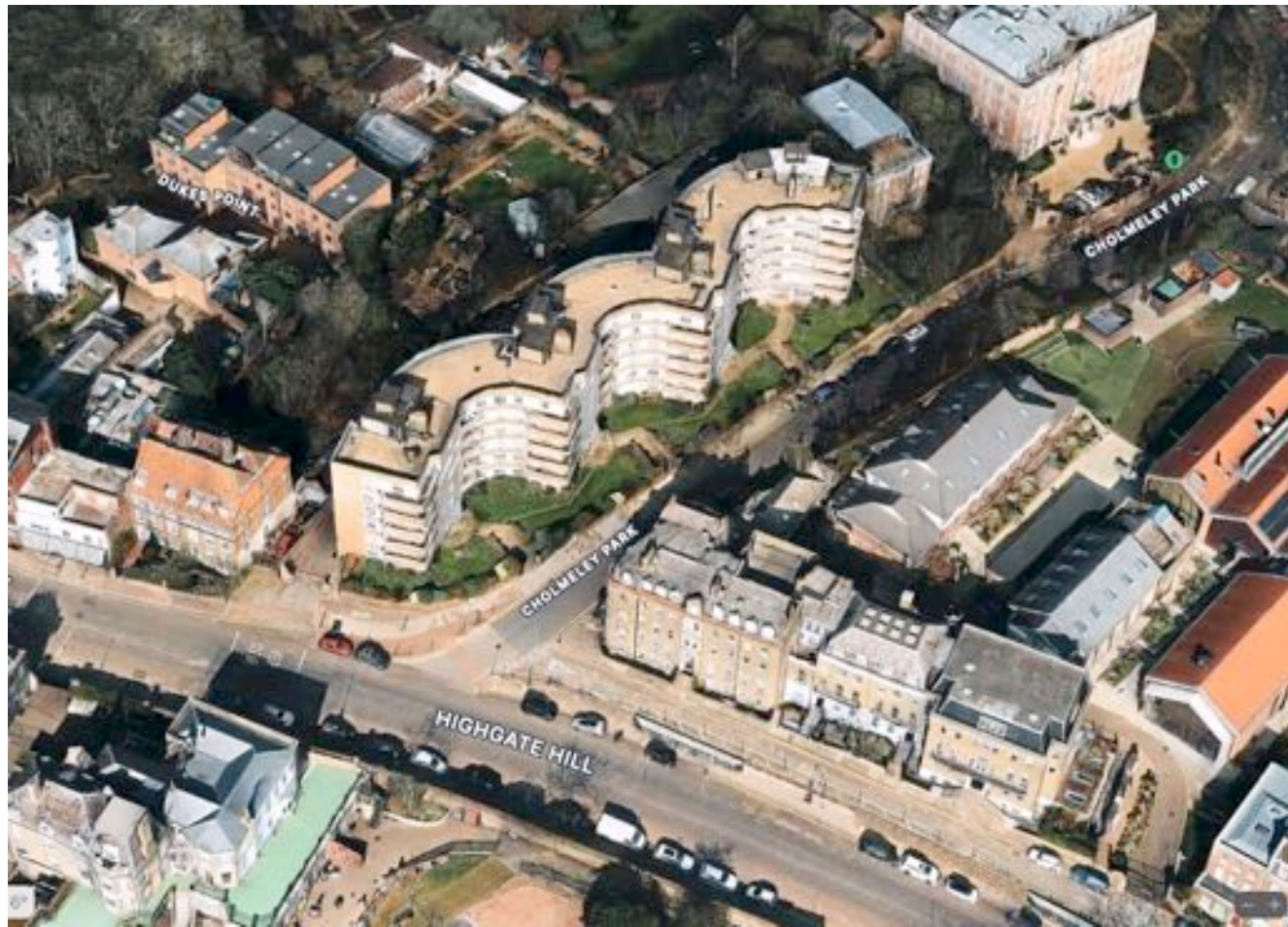
Ariel view looking East
