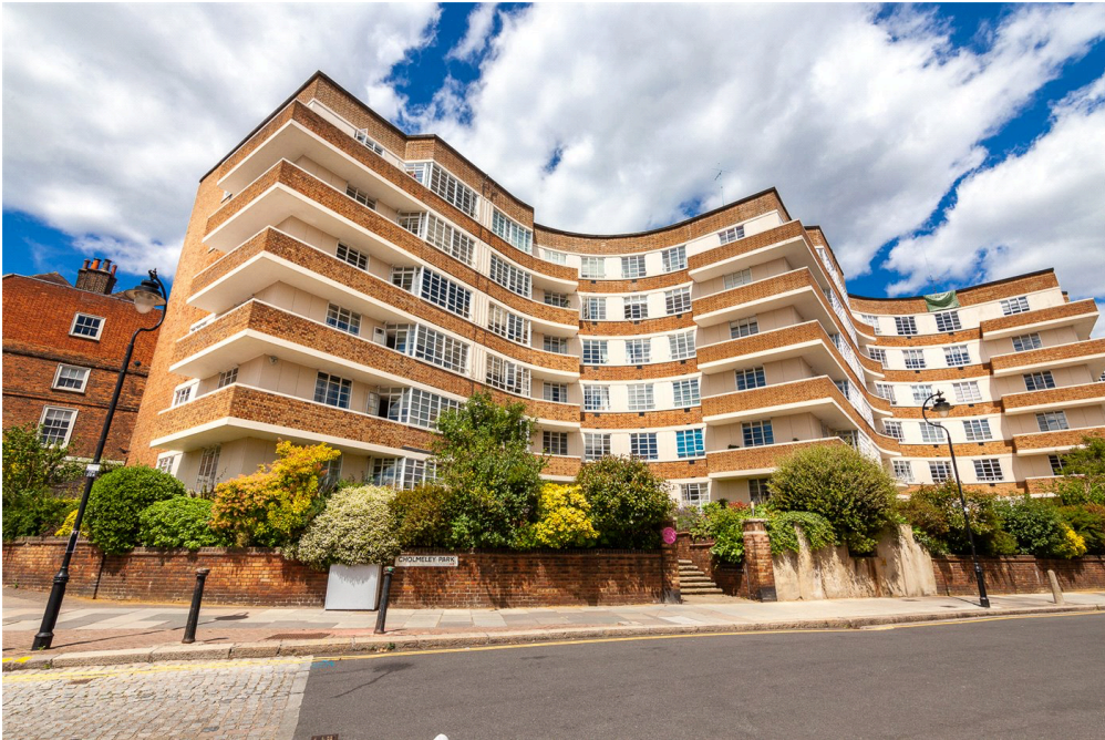
Cholmeley Lodge rooftop guardings
